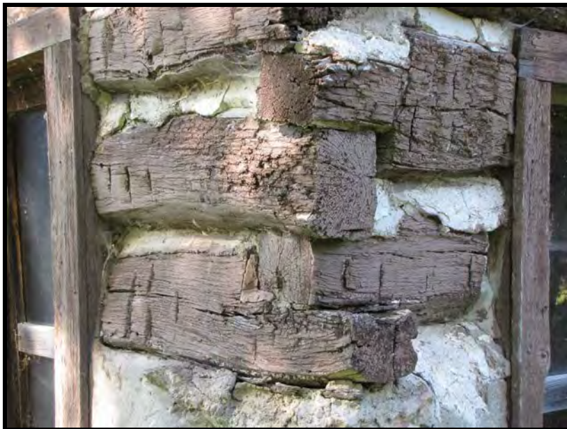
SD_Brookings County_Mortimer Cabin_0007: Log notching detail, South corner, view to North.
