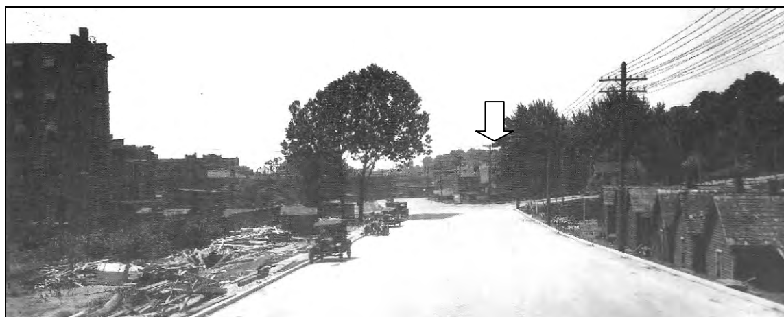
Figure 3. A c. 1929 photograph of Piedmont Avenue under construction; view south toward downtown and State Street. Note worker's housing at right, which became the site of the 1933 United States Post Office, and Hotel Bristol to the left (razed c. 1974). The intersection in the middle of the photograph is Cumberland Street, where the Masonic Lodge would be built in 1931 (arrow location). Credit Tim Buchanan.
