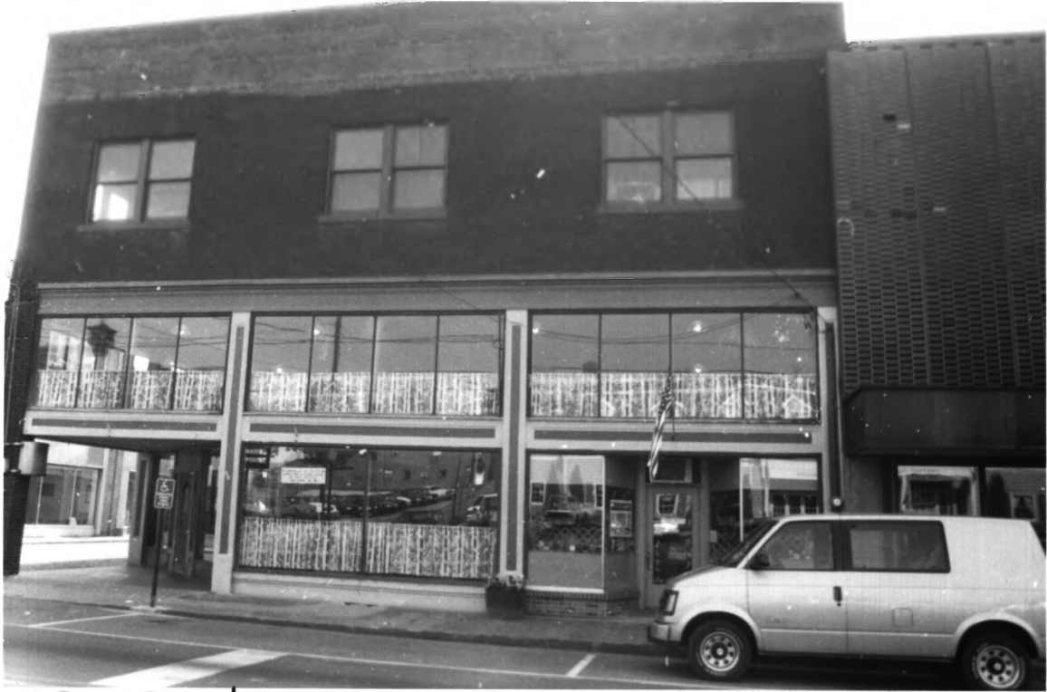
CENTER & ABERNATHY STORE BUILDING POLK CO TN
