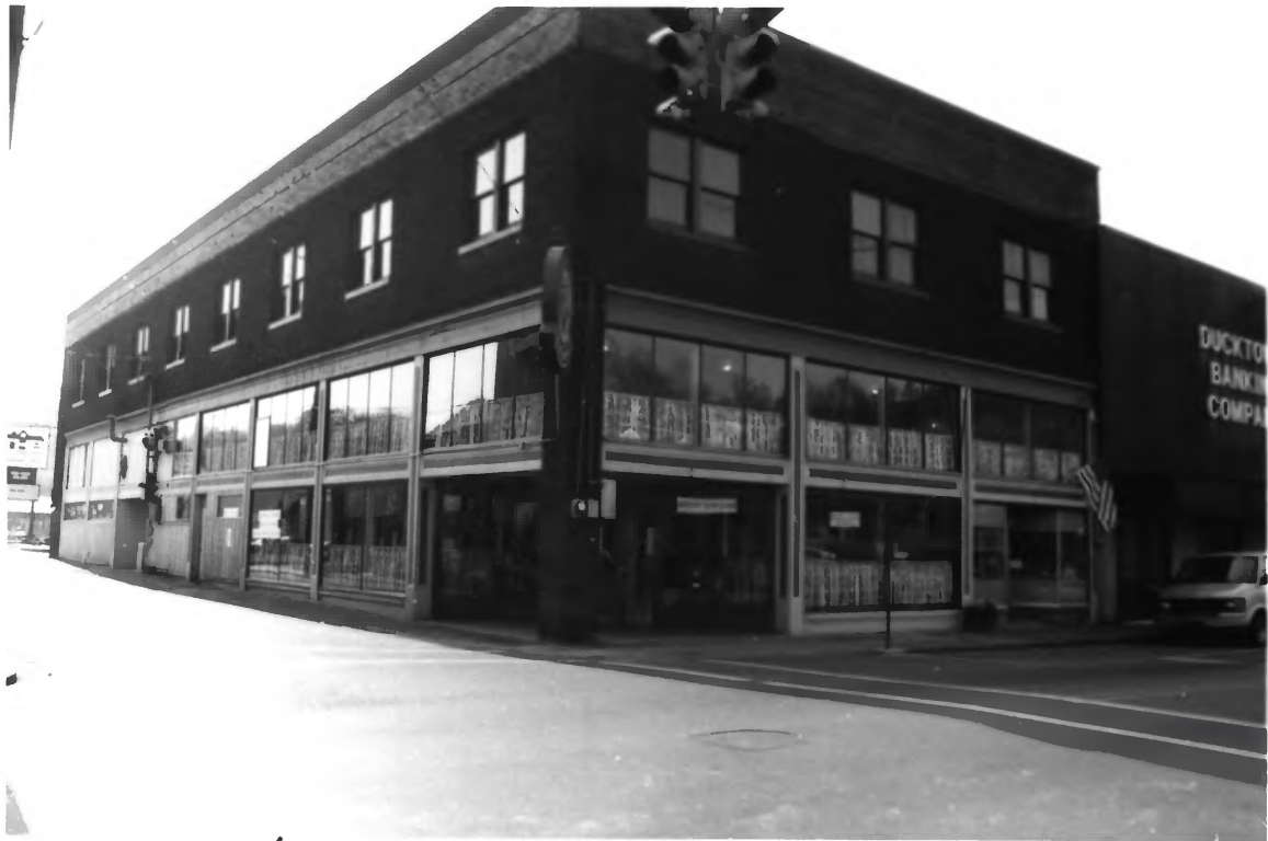
CENTER & ABERNATHY STORE BUILDING POLK CO TN
