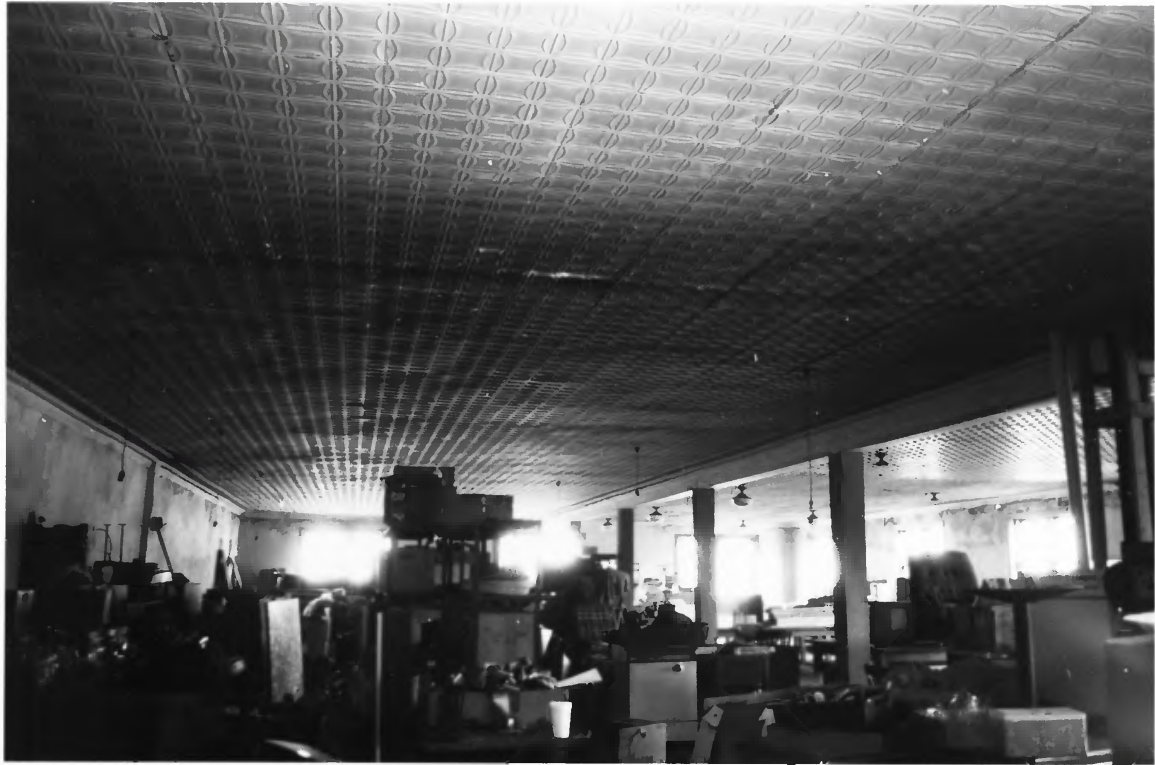
CENTER & ABERNATHY STORE BUILDING POLK CO TN
