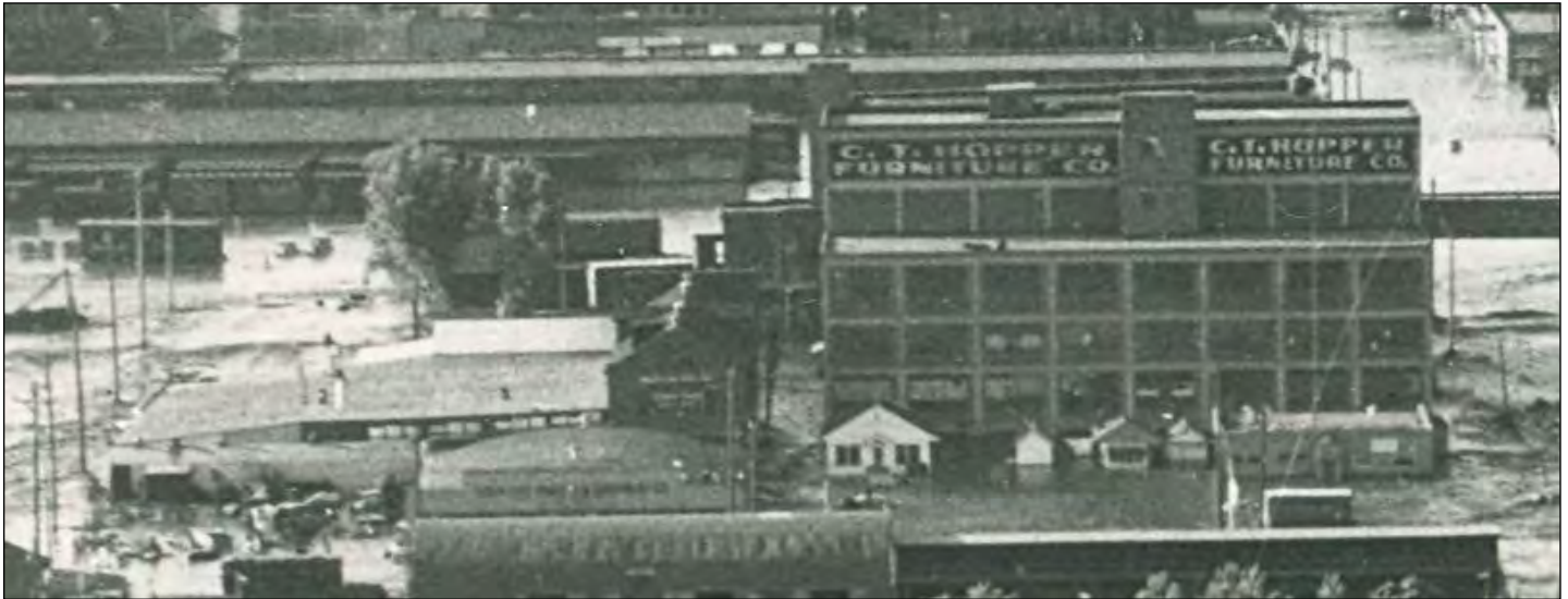
Figure 27: The flooded factory in 1953, looking north from the Missouri River in aerial view (Sioux City Public Museum, SC04.FL.Floyd.1953.072)
