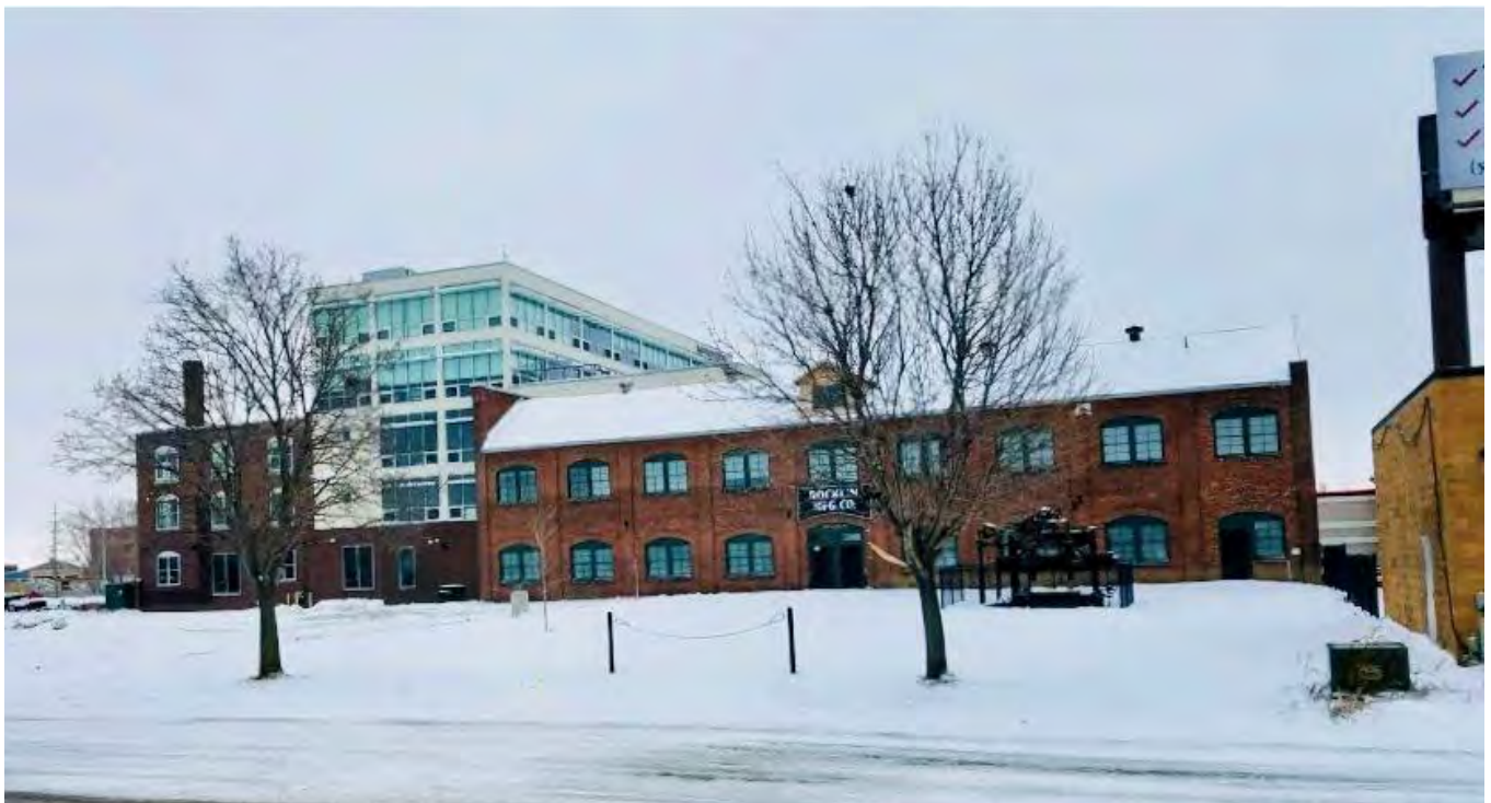
Figure 38: Current building and site appearance, looking northeast (photo by Ross Rocklin, January 2019)
