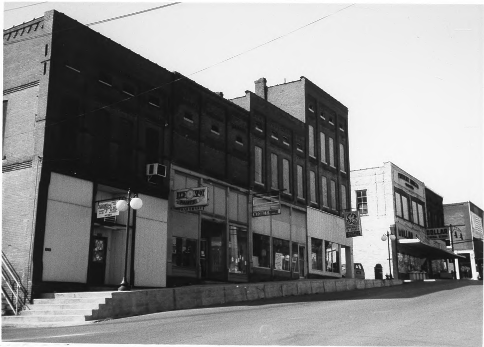
PROVIDENCE COMMERCIAL HISTORIC DISTRICT WEBSTER COUNTY, KY # 5
