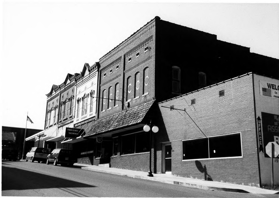
PROVIDENCE COMMERCIAL HISTORIC DISTRICT WEBSTER COUNTY, KY #8
