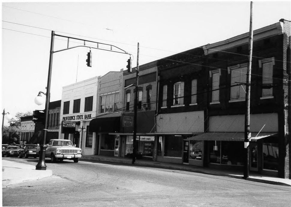
PROVIDENCE COMMERCIAL HISTORIC DISTRICT WEBSTER COUNTY, KY #7
