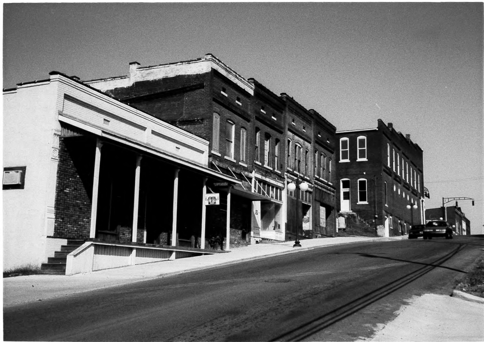
PROVIDENCE COMMERCIAL HISTORIC DISTRICT WEBSTER COUNTY, KY # 9
