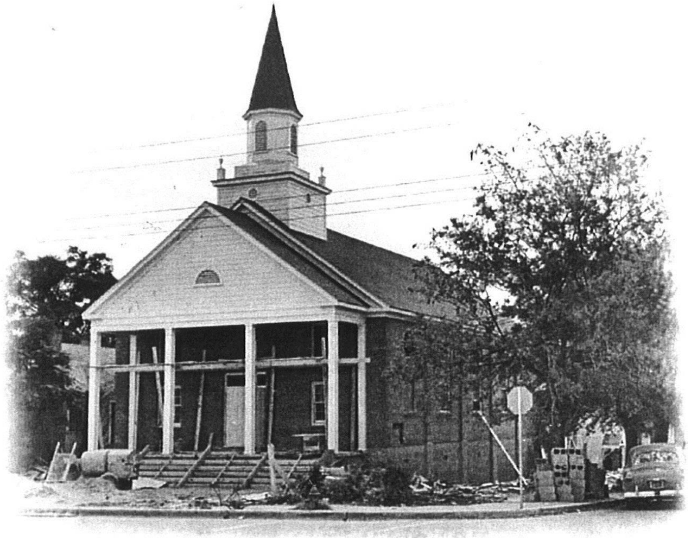
Figure 6: Undated historic photo depicting the church under construction.
