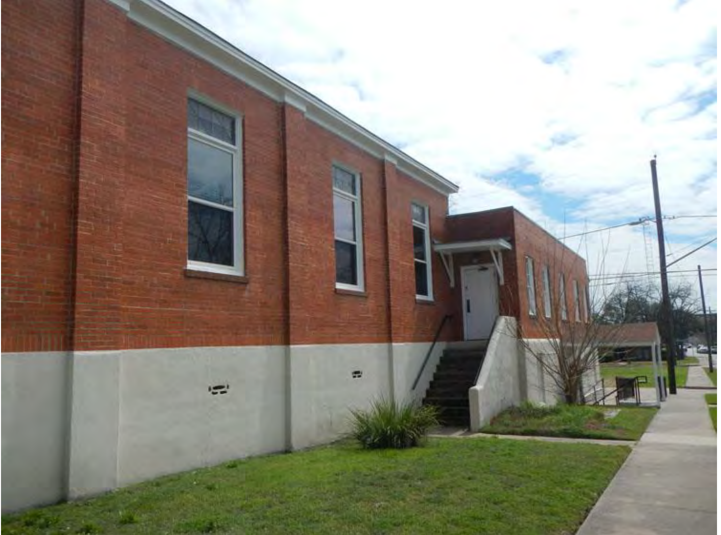
Photo 5: West elevation (partial), camera facing approximately south.
