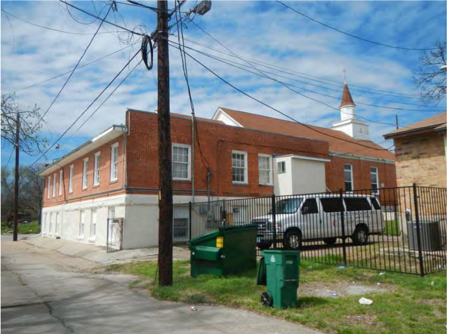
Photo 3: Southeast oblique (partial).
