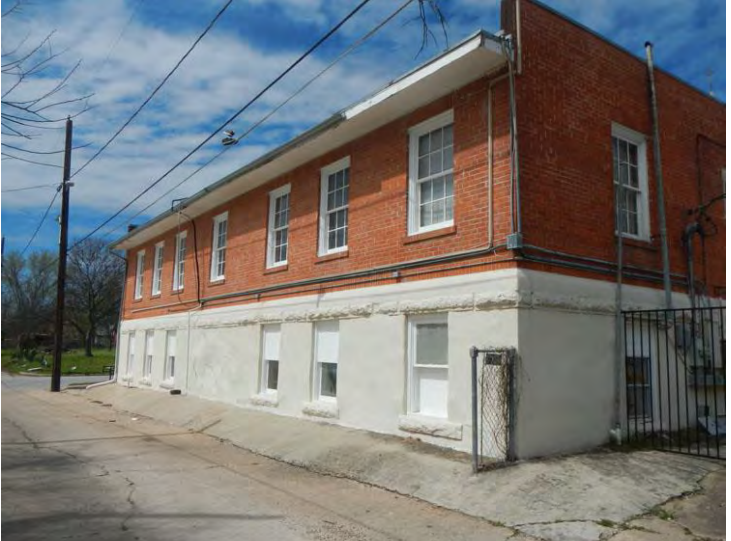
Photo 4: South elevation, camera facing approximately west-northwest.
