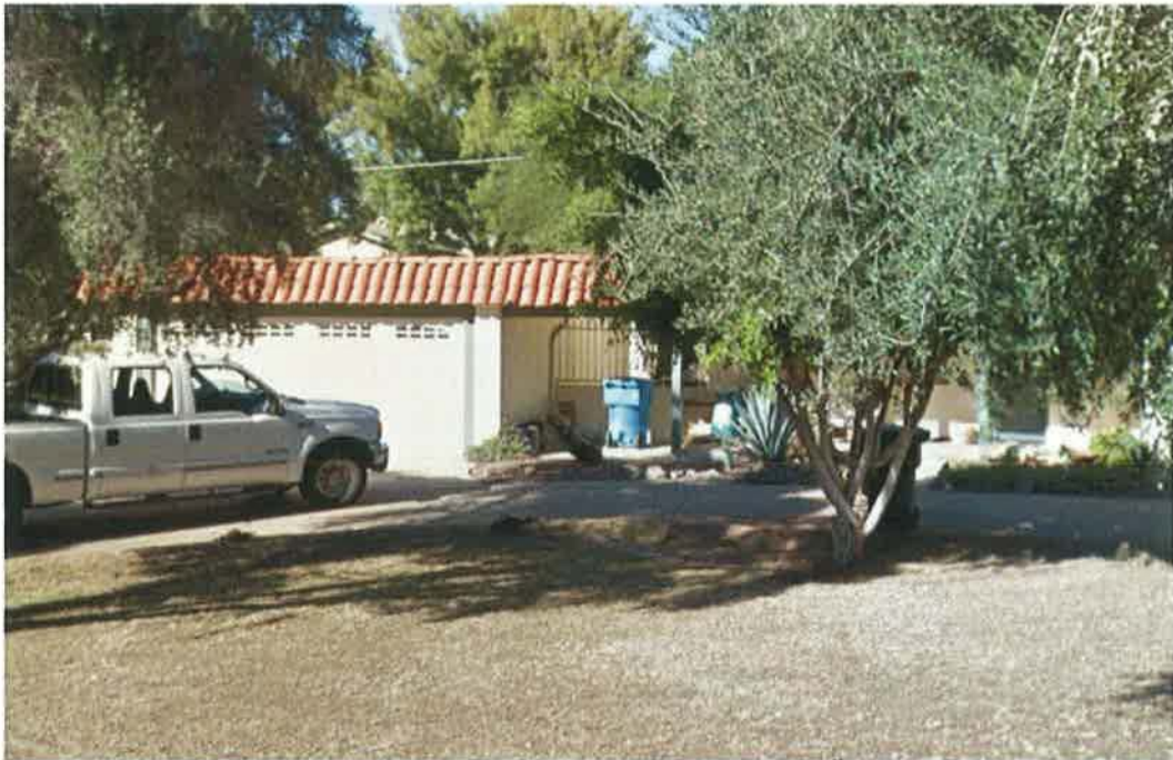
Figure 4. View of the house at 420 E. Oregon Ave. showing the nonhistoric garage detached from the main body of the historic building apart from a connecting roof creating a breezeway. Source: Google, 2016.
