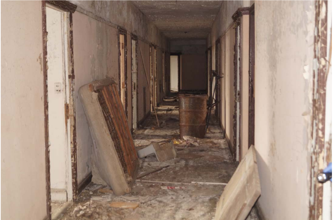
Typical Upper floor Hallway
