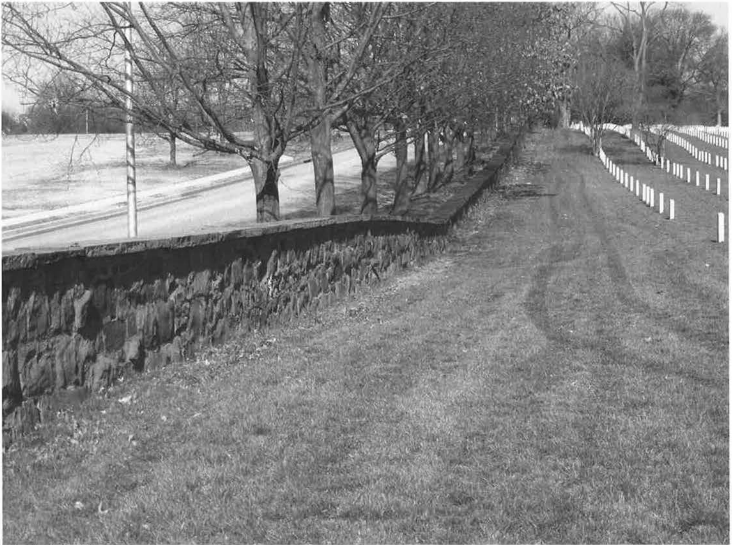
Photo 20. View north along Seneca sandstone boundary wall.
