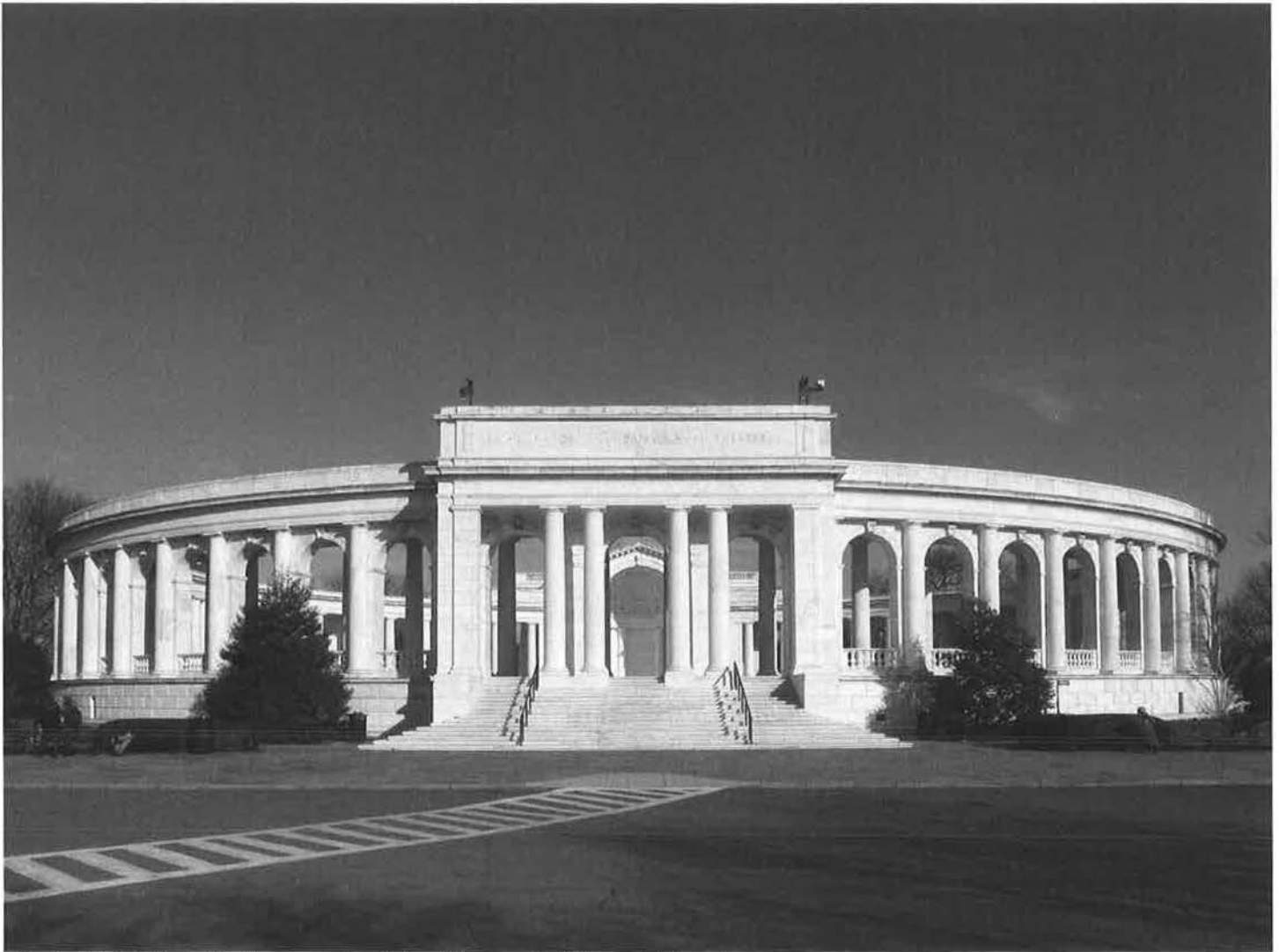
Photo 12. View to the east of the Memorial Amphitheater.
