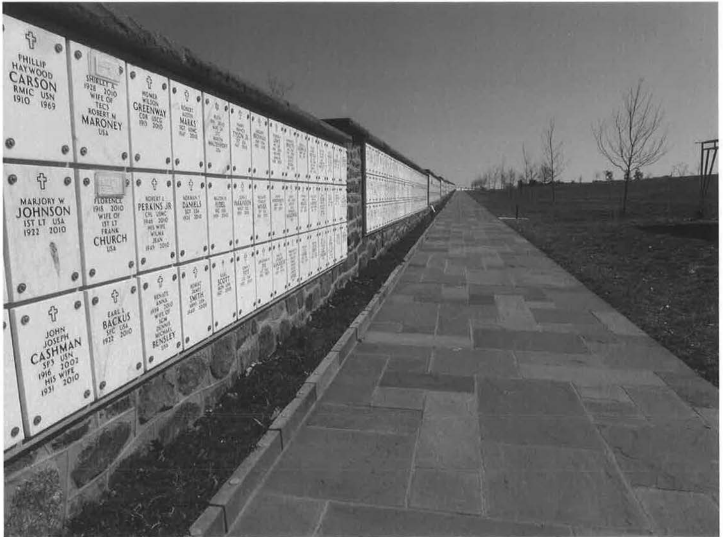
Figure 28. View to the south along the Niche Wall.
