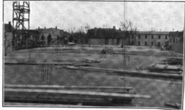
Fig. 3. The First Floor Level, Showing Reinforcing Bars for Columns Extending Above.
