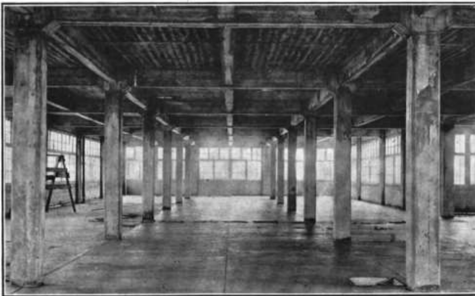
THE FINISHED INTERIOR—SMOOTH CEMENT FLOORS ARE USED THROUGHOUT.
