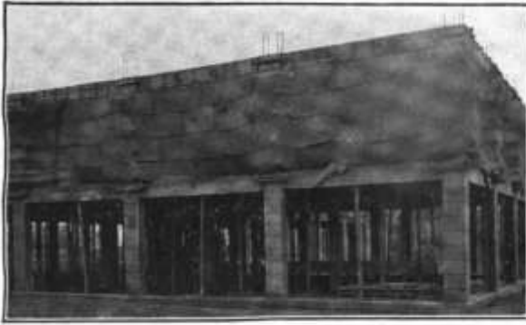
Second Story Enclosed for Protection Against Cold.
