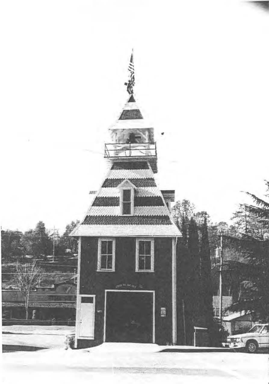
Figure 4 of 4 Historic Fire House No. 2 c 1980
