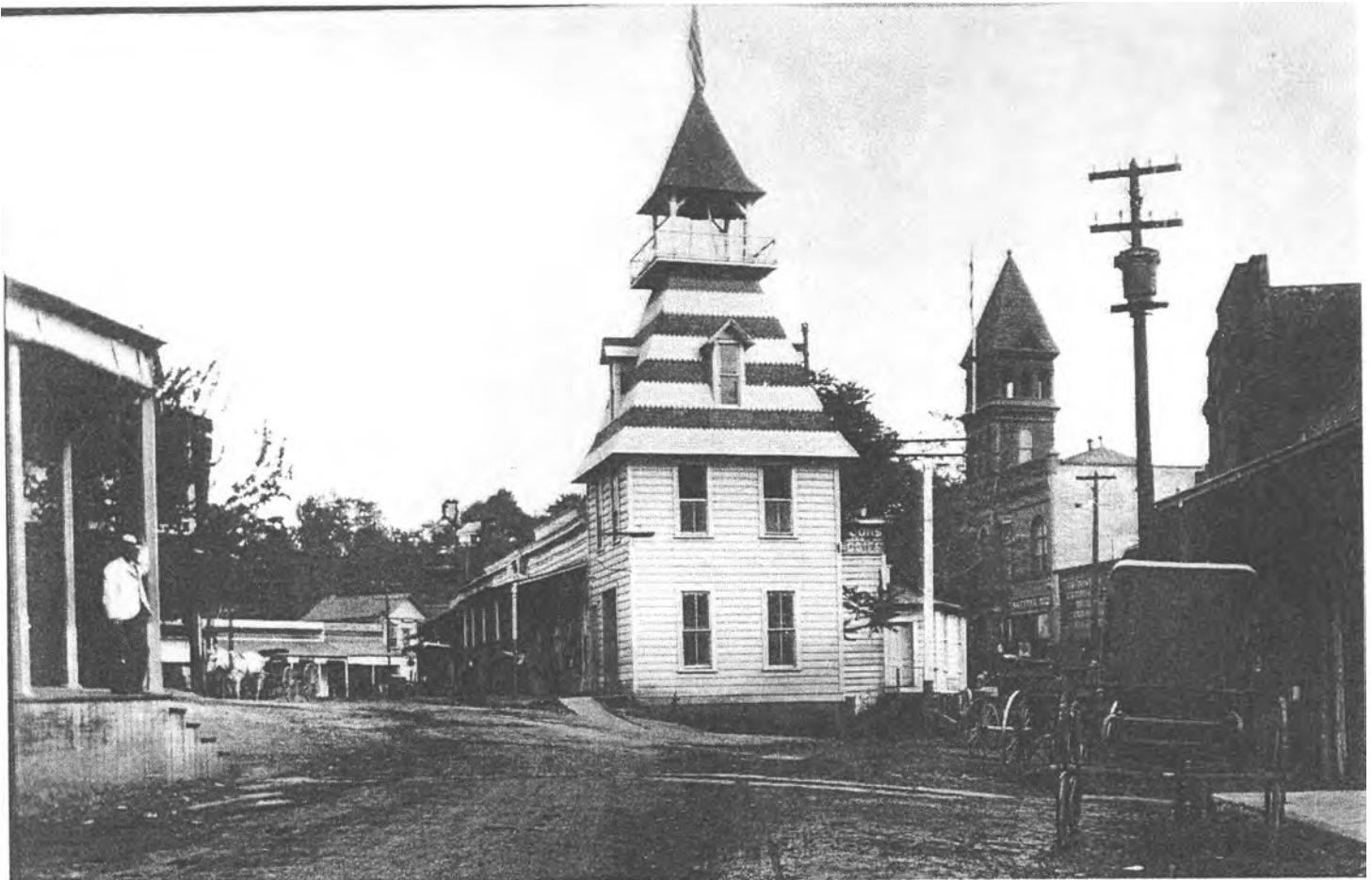
Figure 1 of 4 Historic Fire House No 2 c 1896
