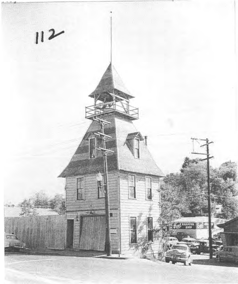
Figure 3 of 4 Historic Fire House No. 2 c.1954
