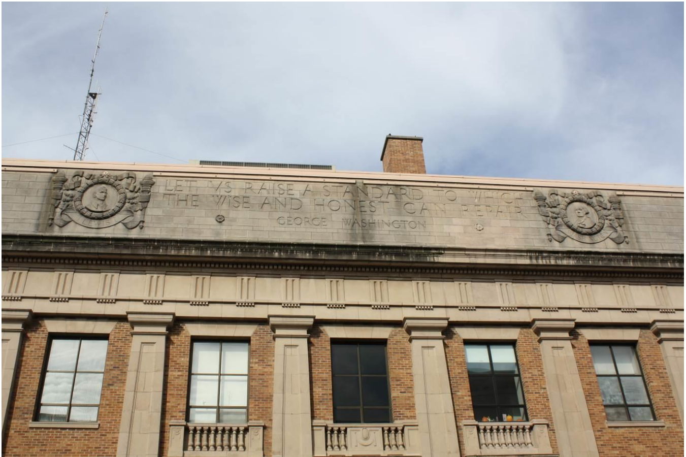
LewisCounty_HistoricCourthouse_007 Cornice Detail – north facade
