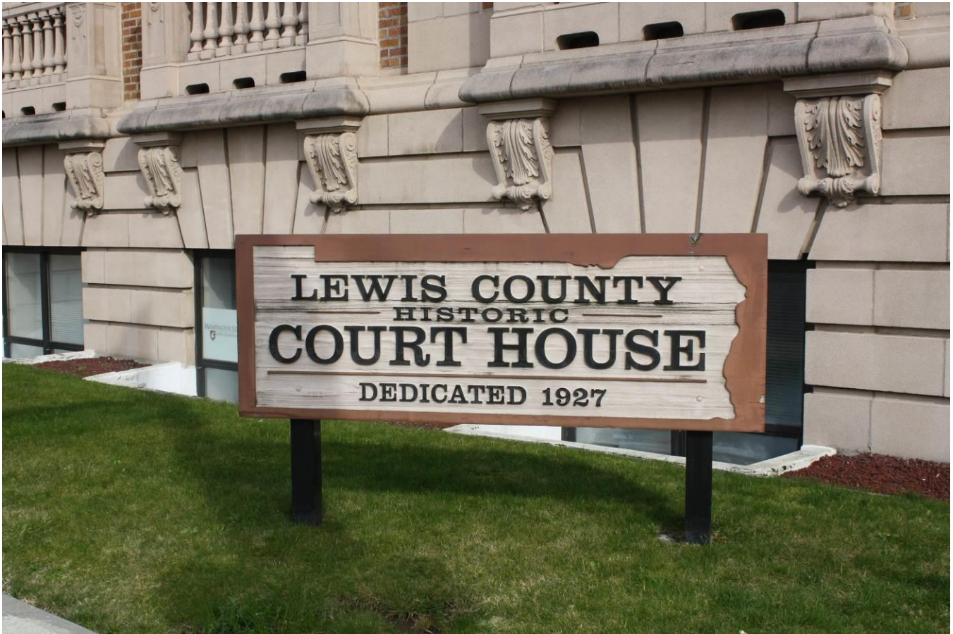
LewisCounty_HistoricCourthouse_005 Window sill detail
