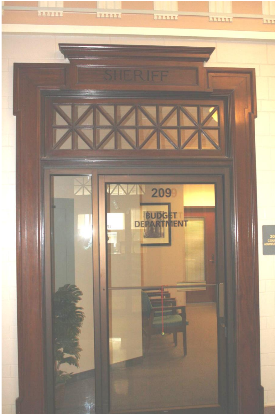
LewisCounty_HistoricCourthouse_016 Second floor office door detail
