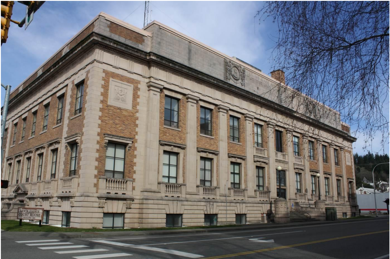
LewisCounty_HistoricCourthouse_004 South (Main Entry) Facade
