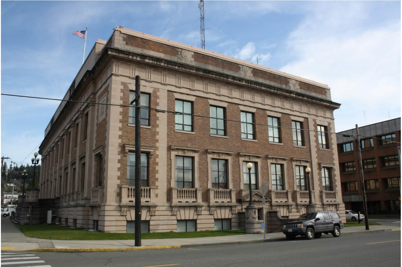
LewisCounty_HistoricCourthouse_003 West facade
