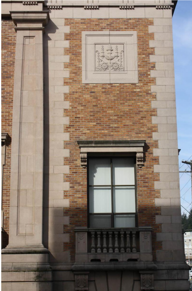
LewisCounty_HistoricCourthouse_009 Facade Detail – SE corner
