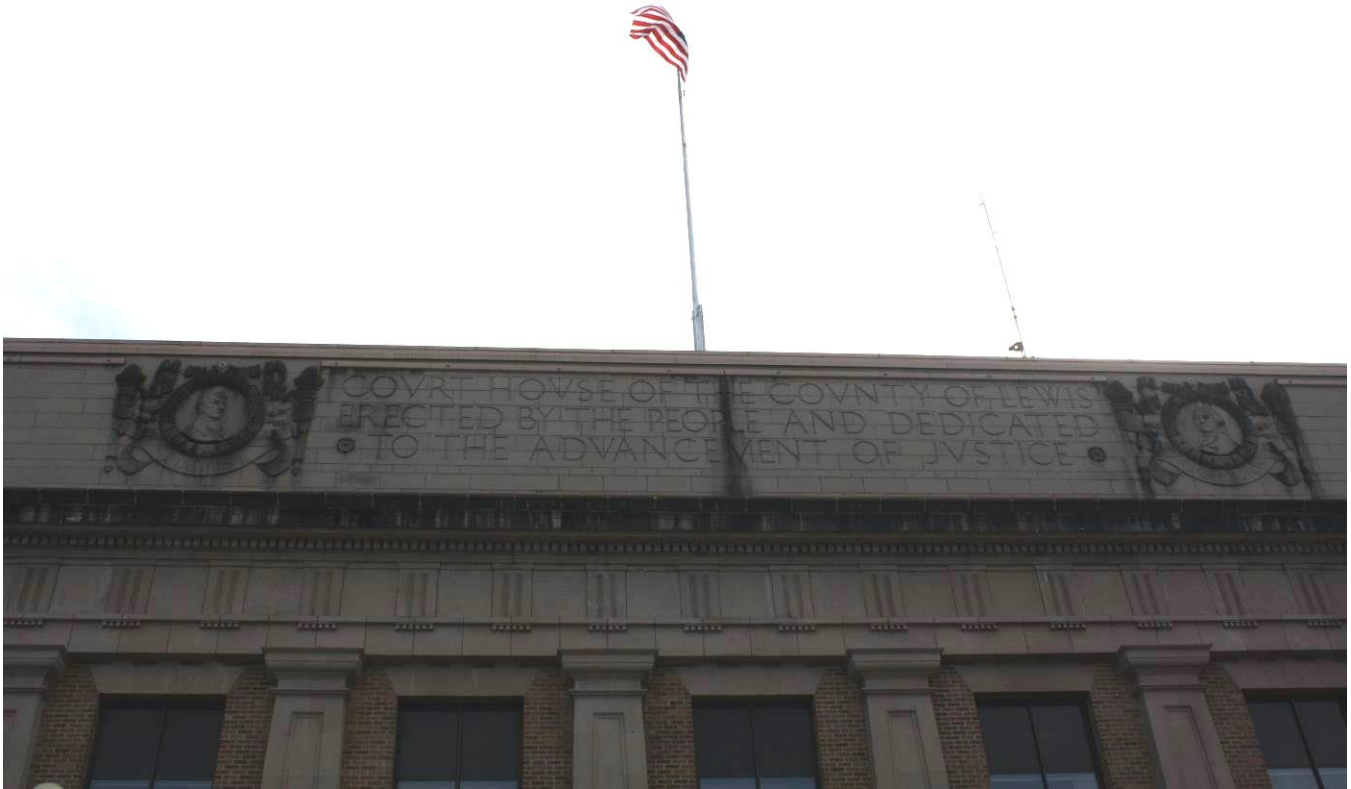
LewisCounty_HistoricCourthouse_006 Cornice Detail – south facade
