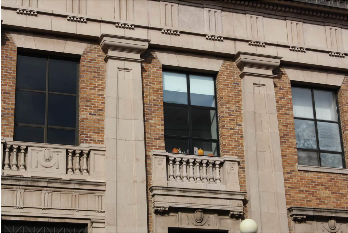
LewisCounty_HistoricCourthouse_008 Detail – south façade (former sky bridge entry point)
