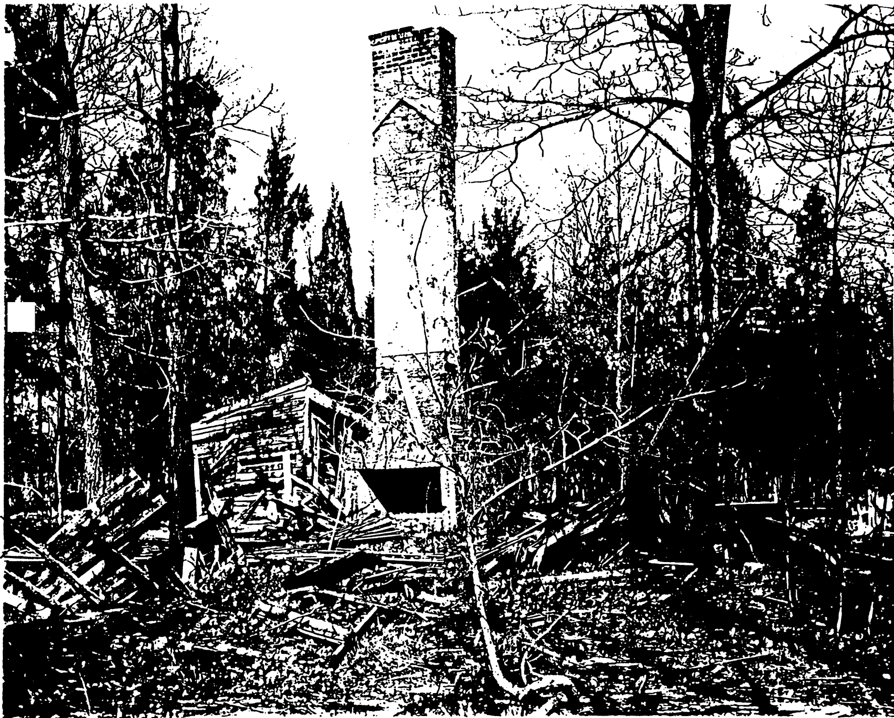
Estellville Glassworks Historic District, Estell Manor City, Atlantic County, New Jersey Workers Houses Site (Site #6) ca. 1980's
