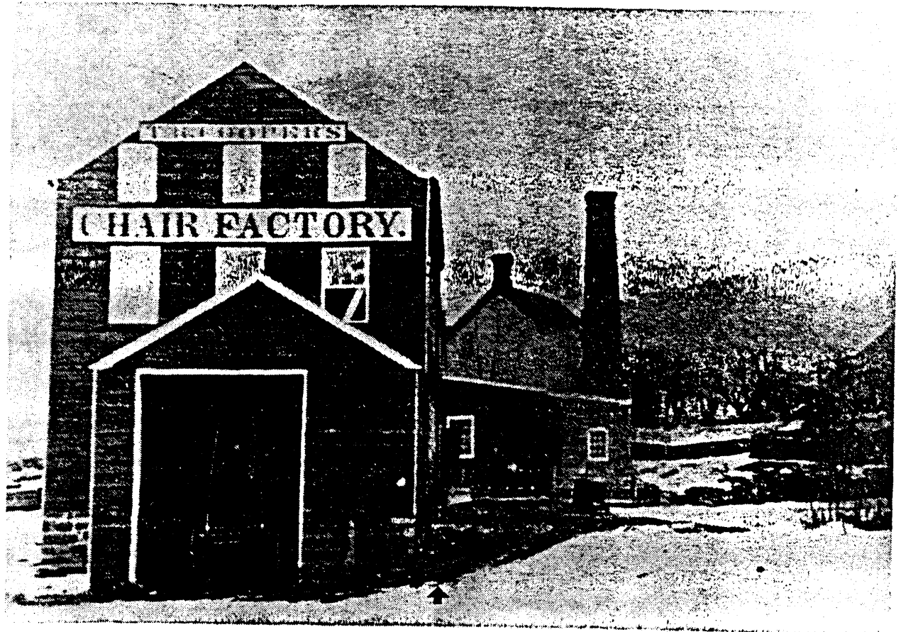
Plate 1. The west facade of the Tunis R. Cooper chair factory ca. 1880. Note chimney and compare with Plate 7. Also note rock platform along the southern foundation wall (arrow), apparently constructed to level the embankment, and the post in the foreground. Evidence for both features was found in excavation (Photo courtesy of Betty Schmelz).
