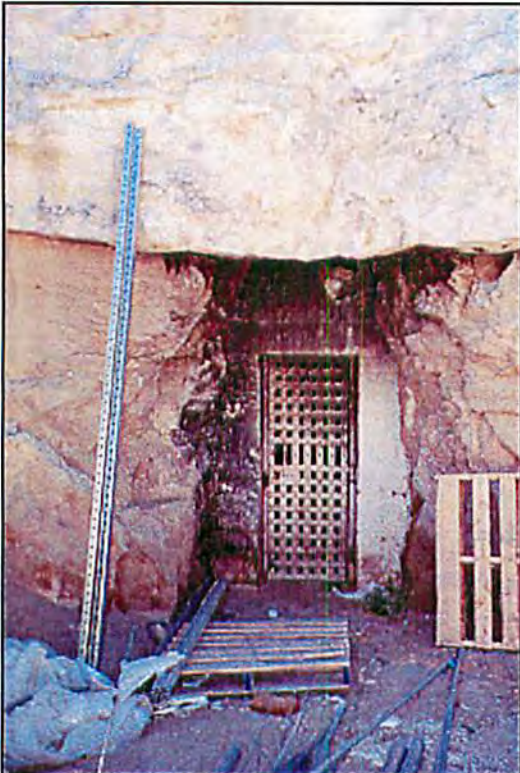
Lockdown cell in quarry, view to west
