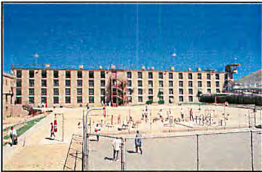
The Yard, with Cell Block A at left, Cell Block B at right, view to east
