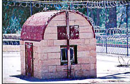
Pump House, view to southwest
