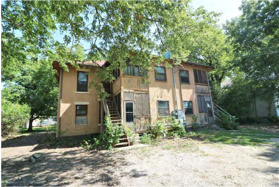
03: South/rear façade with former porches enclosed – The Avalon, taken July 2018
