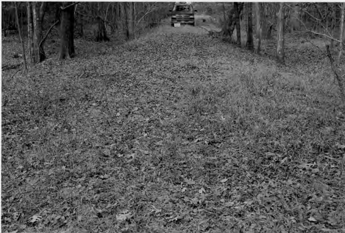
50. Example of a Tram Road Bed, facing north Middleton Place 4300 Ashley River Road Dorchester County, South Carolina Photograph by Lissa Felzer 12/13/2007
