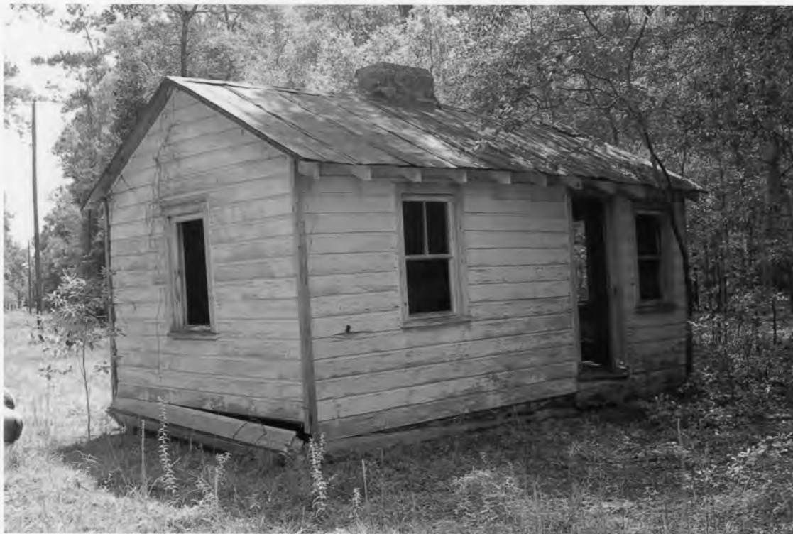
65. Cabin (Inventory 18t), northwest elevations Millbrook Plantation Ashley River Road Charleston County, South Carolina Photograph by Lissa Felzer, 8/21/2008
