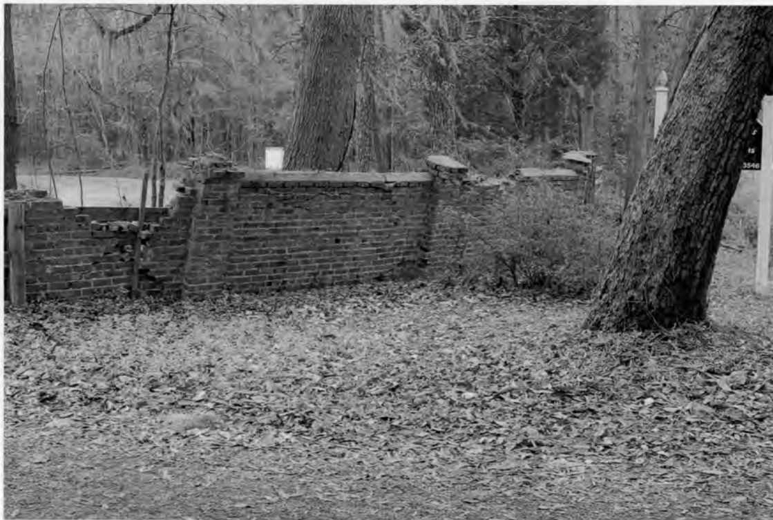
23. Entrance Wall, facing south Wragg Plantation/ Mateeba Gardens 151 Mateeba Gardens Road Dorchester County, South Carolina Photograph by Lissa Felzer, 3/2/2008
