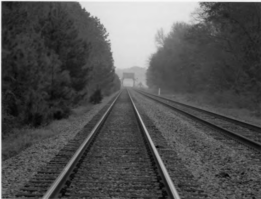
97. Railroad Trestle, facing south Ashley River Road Charleston County, South Carolina Photograph by Christina Shedlock, 3/22/2010
