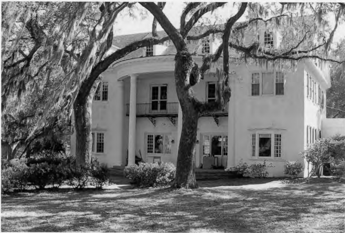
57. Carter House, north elevation Millbrook Plantation Ashley River Road Charleston County, South Carolina Photograph by Lissa Felzer, 3/2/2008
