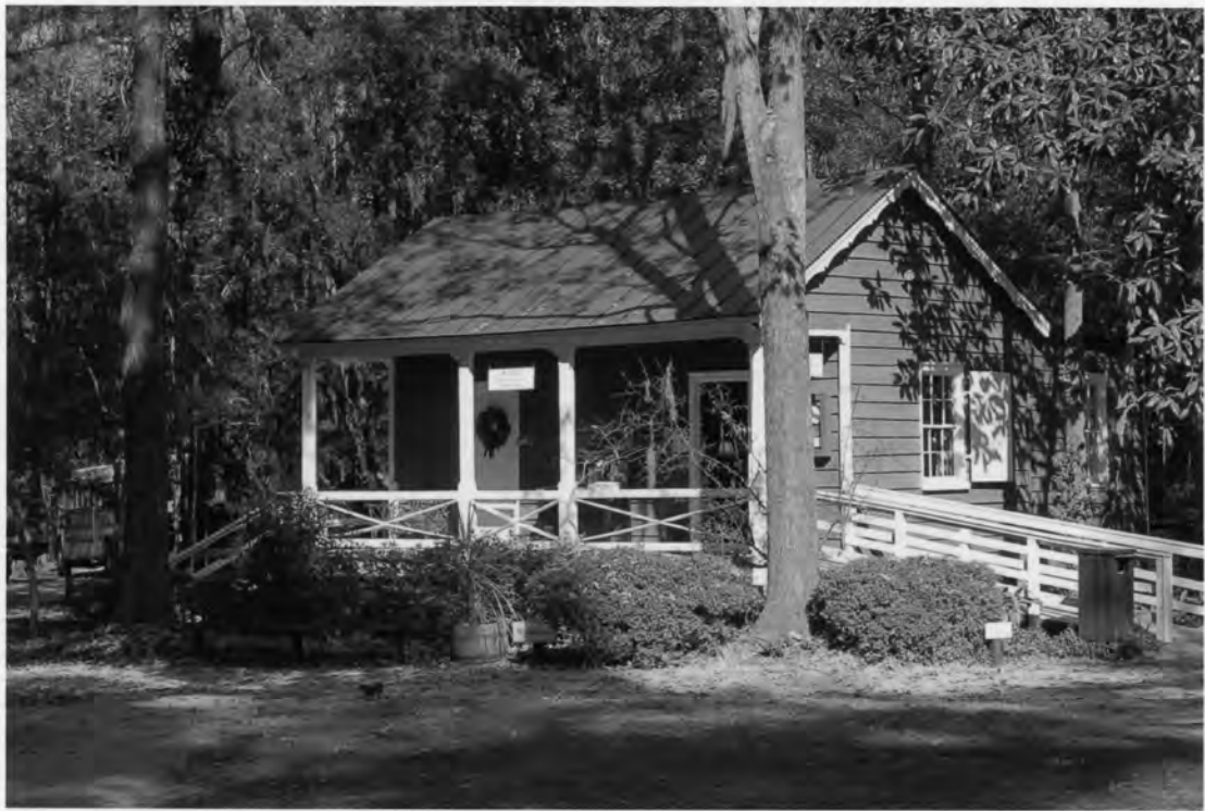
86. Caretaker's Residence, facing northeast Drayton Hall 3380 Ashley River Road Charleston County, South Carolina Photograph by Lissa Felzer, 12/10/2007
