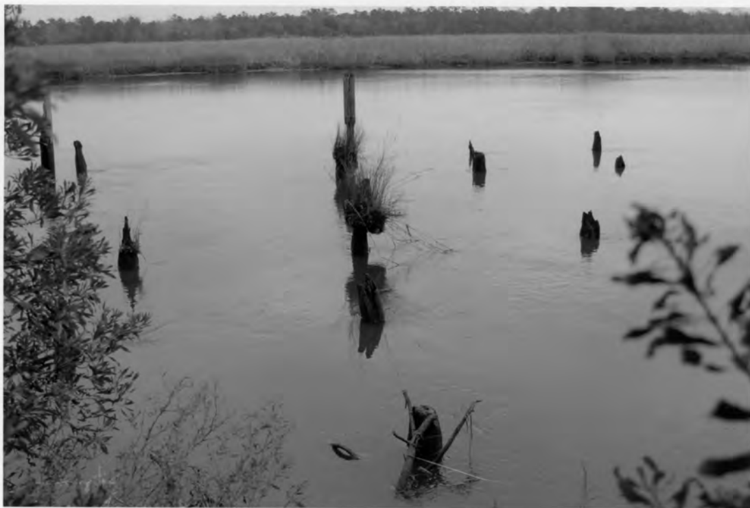
32. Wharf Structure Remnants, facing northeast Uxbridge Plantation Ashley River Road Dorchester County, South Carolina Photograph by Lissa Felzer, 1/26/2009
