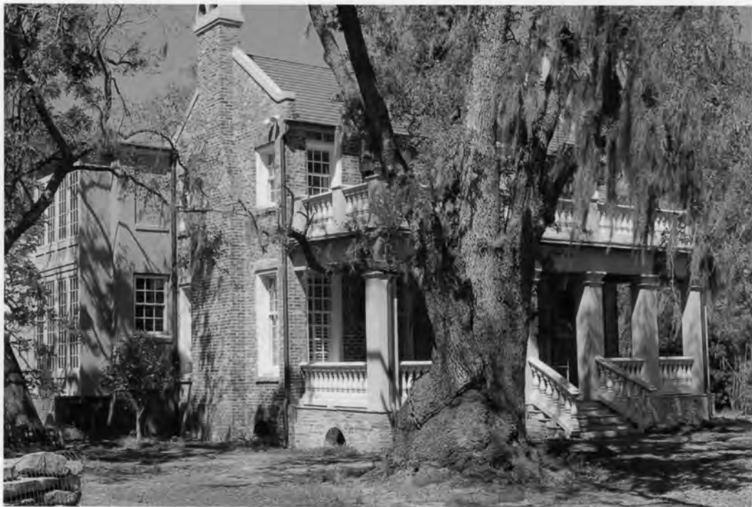
18. Main House, East and South elevations Haggard Hall/The Laurels 295 O'Sullivan Lane Dorchester County, South Carolina Photograph by Lissa Felzer, 4/17/2008
