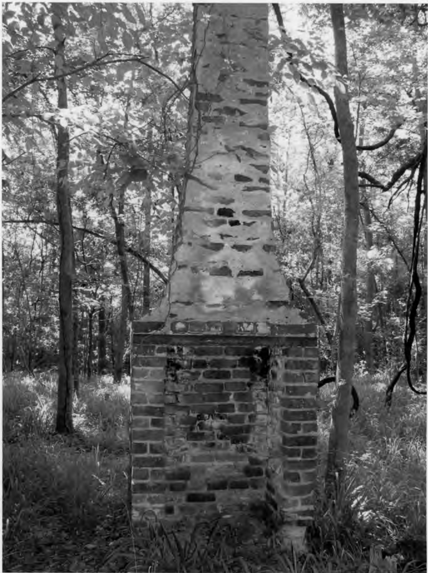
92. MacBeth Road and Associated House Sites, Drayton Hall Chimney at the Roberts-McKeever House Site Charleston County, South Carolina Photograph by Lissa Felzer, 5/31/2008
