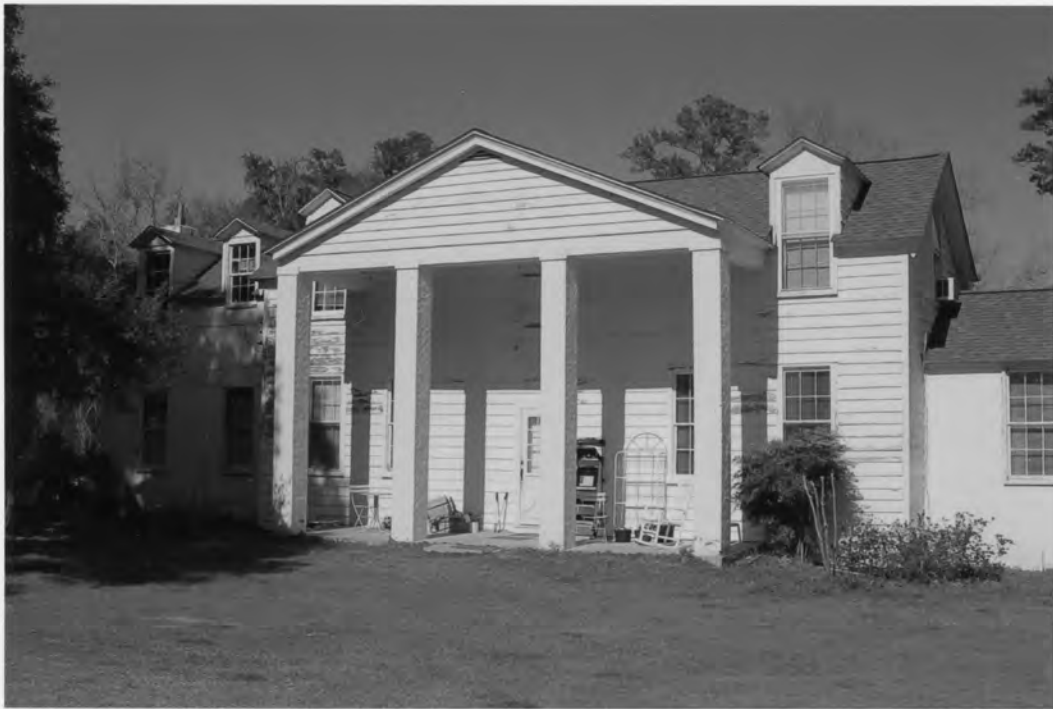
19. Late-19th-century Plantation House Wragg Plantation/Mateeba Gardens 151 Mateeba Gardens Road Dorchester County, South Carolina Photograph by Lissa Felzer, 3/2/2008
