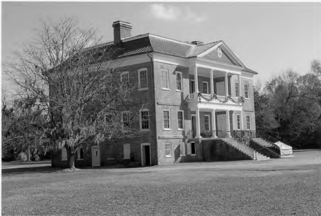
79. Drayton Hall, south and west elevations Drayton Hall 3380 Ashley River Road Charleston County, South Carolina Photograph by Lissa Felzer, 12/10/2007
