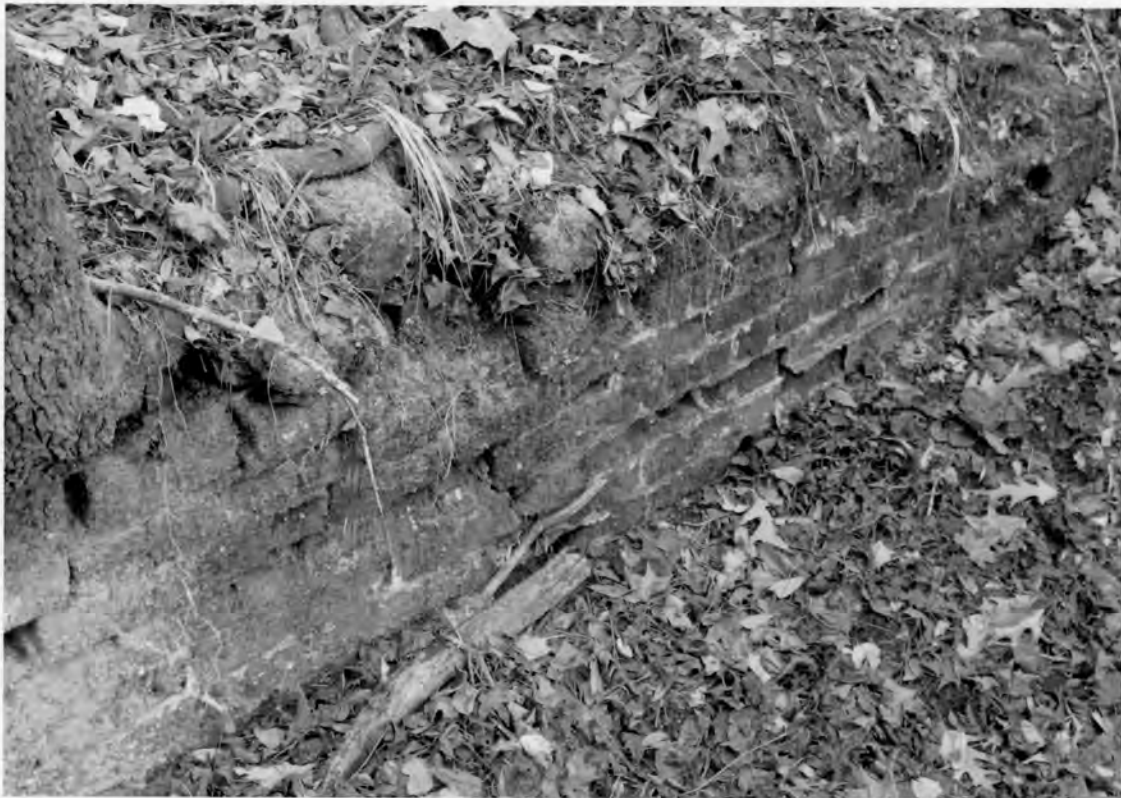
51. W. Cattell Site # 1, detail of brick Middleton Place 4300 Ashley River Road Dorchester County, South Carolina Photograph by Andrew Agha 1/28/2008
