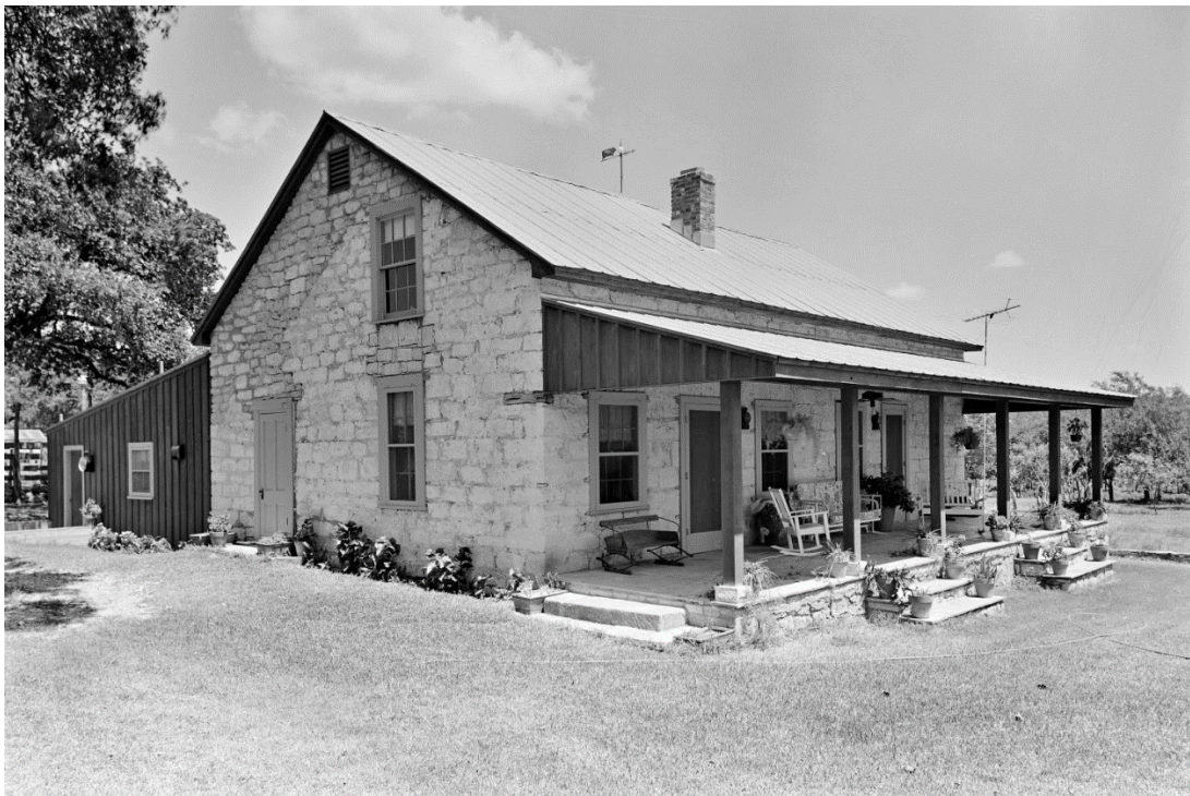
Figure 5. Survey Photo: August 18, 1975. Note historic changes to limestone visible on west elevation to accommodate alterations to roof form. On file at Texas Historical Commission.
