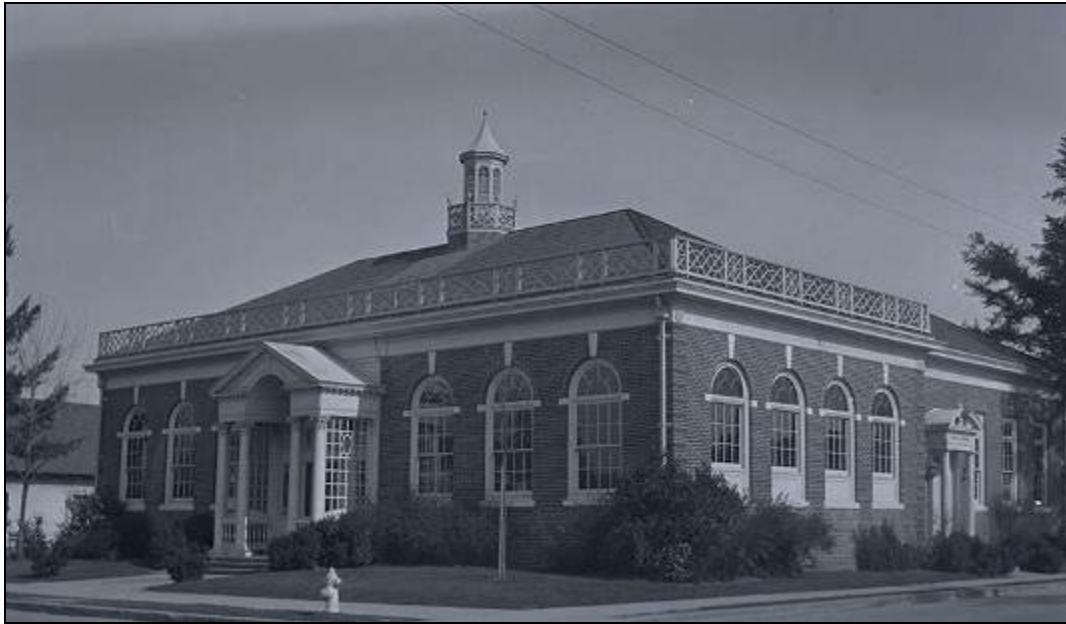
Figure 23: Circa 1920 view southwest corner of Arleta Branch Library, looking northeast. Photo courtesy of Multnomah County Library.
