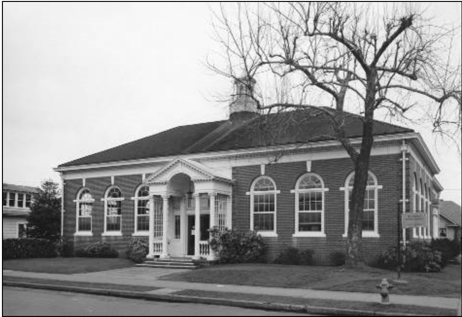
Figure 29: 1963 view of front (west) elevation of Arleta Branch Library. Photo courtesy of Multnomah County Library.
