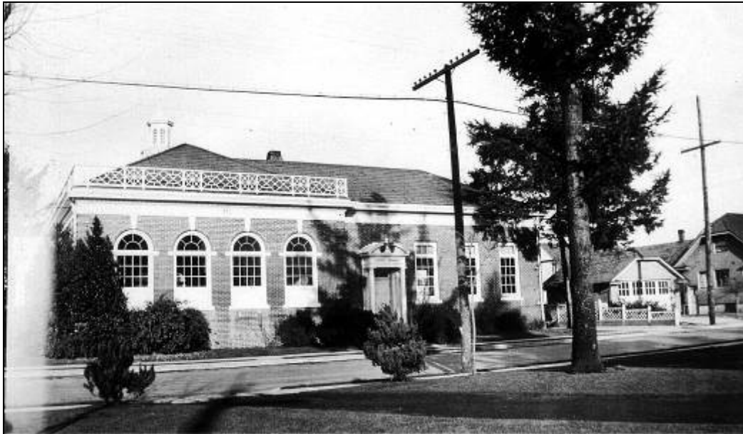
Figure 25: 1923 view of south side elevation of Arleta Branch Library, looking north/northeast. Photo courtesy of Multnomah County Library.
