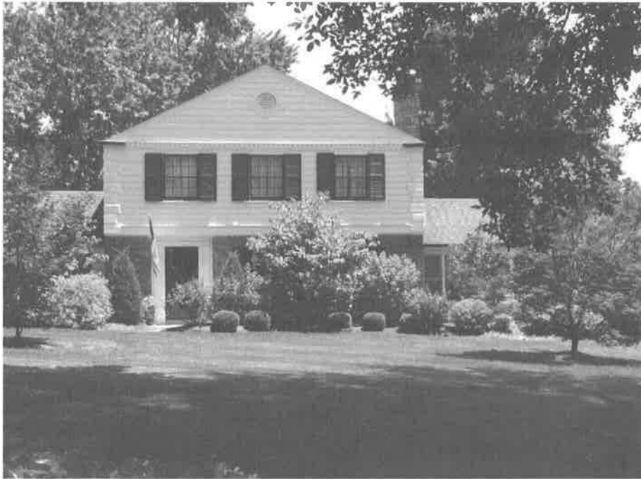
Figure 9: The house at 8 Berkley Lane (1938; George A. Winkler). (Source: Preservation Research Office photograph, 2013.)
