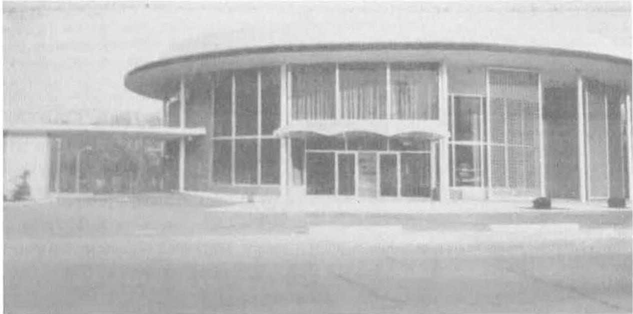
Figure 6: First Security Bank (1961; Rathert & Roth). (Source: St. Louis Construction Record .)
