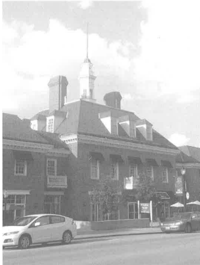
Figure 11: The Reliance Life Insurance Company Building (1963; Winkler & Thompson). (Source: Preservation Research Office photograph, 2013.)
