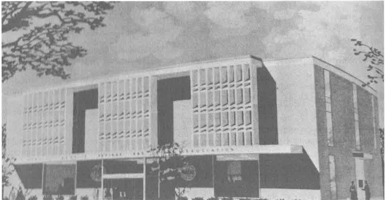
Figure 7: Public Service Savings and Loan Association Building (1962; Kenneth Wischmeyer). (Source: St. Louis Construction Record .)
