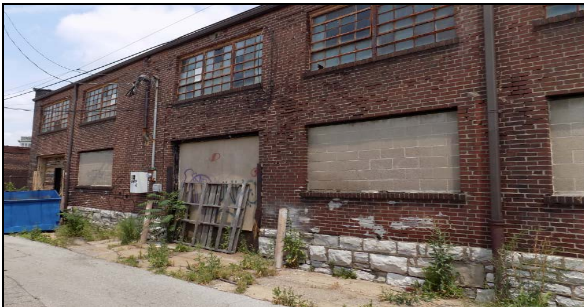
Figure 14: Rear, south-facing elevation of the building. Loading dock at far left side is original to the building's design; the garage bay near the center was added by Bradshaw for Frier-Sturgis in 1926. Source: Matt Bivens, 6-2016.
