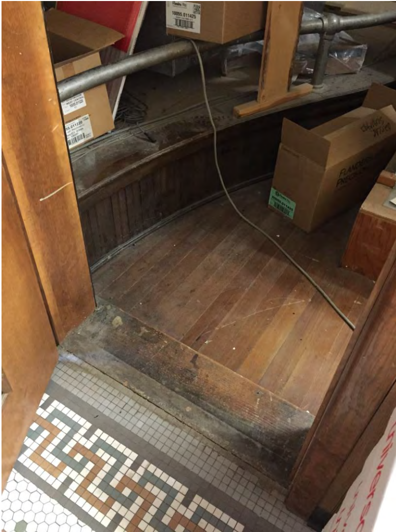
Photo 21 Third floor mezzanine level.
