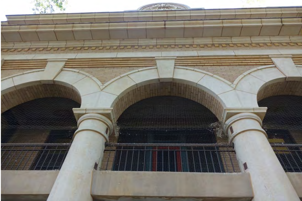
Photo 6 Second floor balcony, west side.
