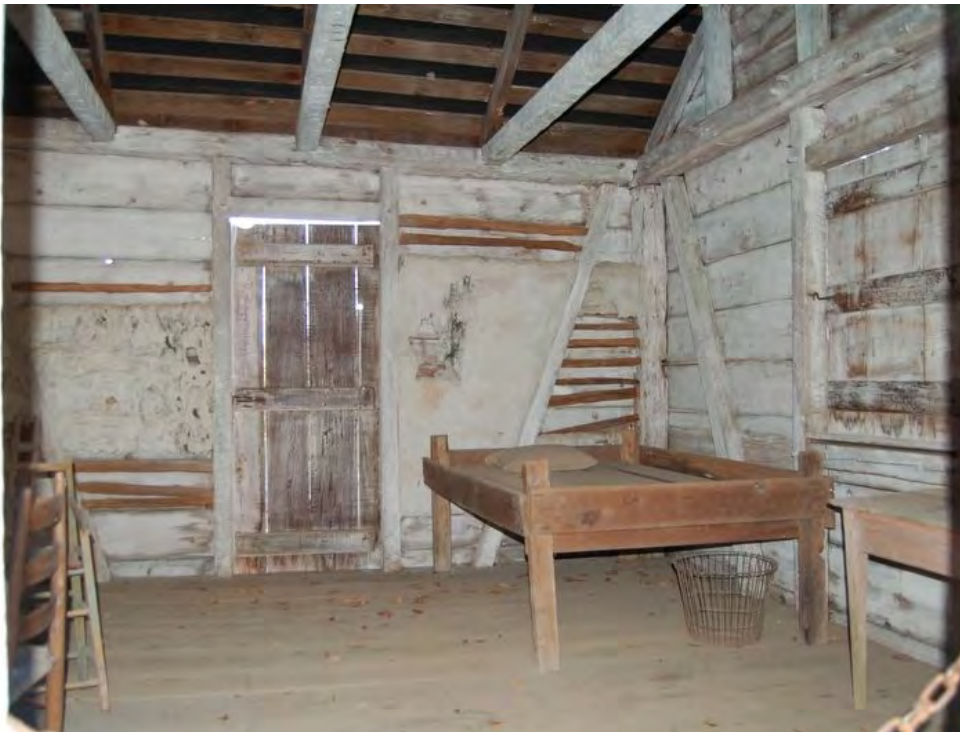
Figure 16: Interior of Tyrone slave cabin at the LSU Rural Life Museum, from HMdb.org (The Historical Marker Database) Note that the cabin is constructed of both bousillage and briquette entre poteaux (brick between post).
