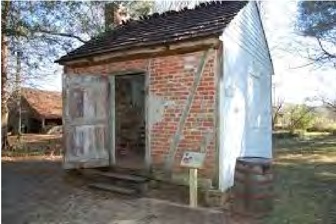
Figure 16: Interior of Tyrone slave cabin at the LSU Rural Life Museum, from HMdb.org (The Historical Marker Database) Note that the cabin is constructed of both bousillage and briquette entre poteaux (brick between post).
