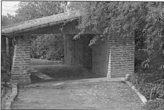
Photograph #13 Carport, camera facing southwest.
