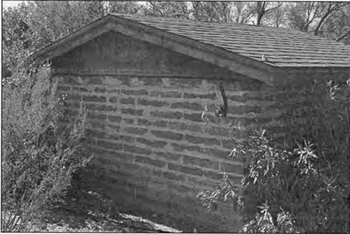
Photograph #21 Well house, camera facing southwest.
