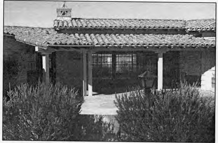
Photograph #6 North façade, front porch detail, camera facing southwest.
