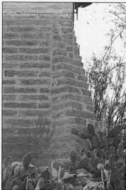
Photograph #11 Buttress at southwest corner, camera facing southeast.
