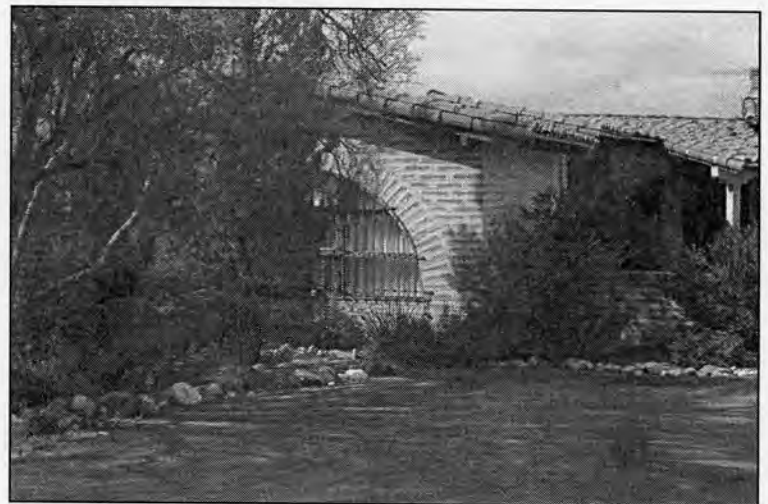
Photograph #12 Northeast projecting service wing, 1964 addition, camera facing south.
