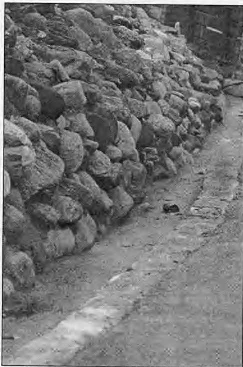
Photograph #3 Cobble masonry retaining wall with concrete drainage detail along secondary drive, camera facing south.
