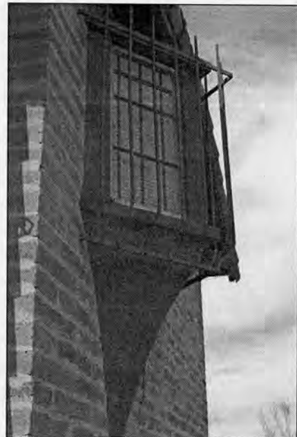
Photograph #10 Oriel window on upper bedroom, west facade, camera facing southwest.
