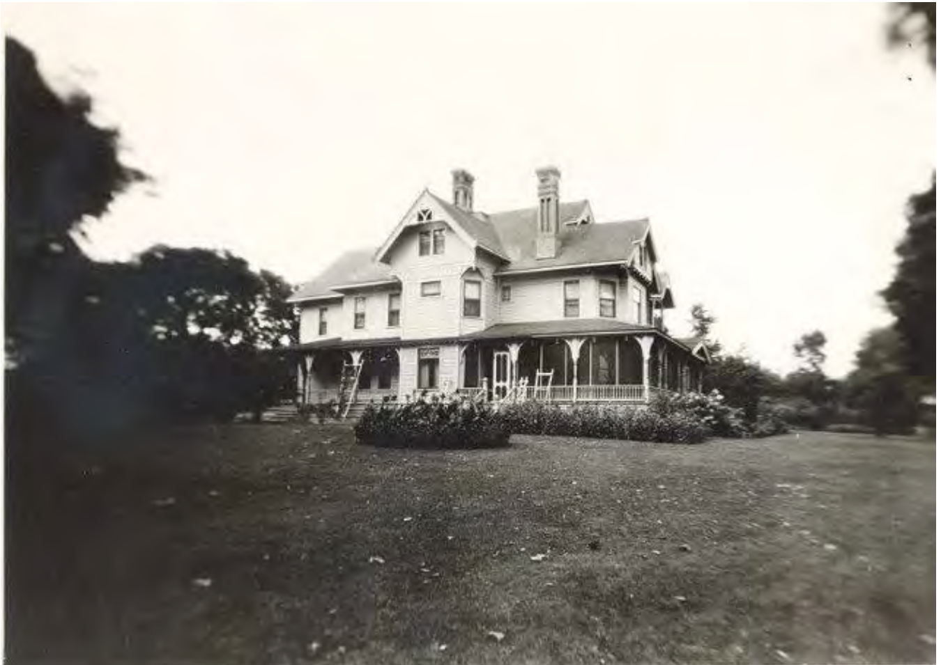
Figure 13: Pre-1947 view of the Johnson House looking northwest showing screened-in veranda.
