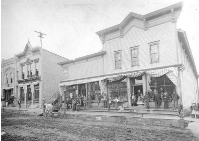
Figure 32: Johnson, Hill & Company store (right), 1890s.
