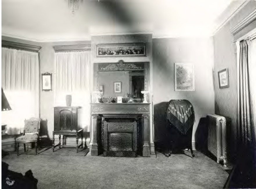
Figure 18: Fireplace in front parlor, 1947.
