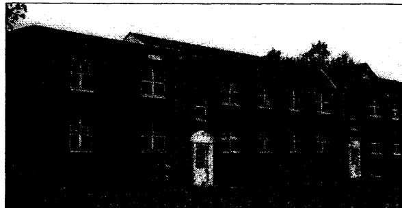
Figure 7-2. Contrast of roof lines within one building, looking northeast to Building 4455.
