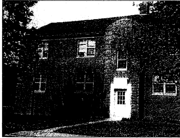
Figure 7-4. Entry detail, I-shaped building at 4500 Marcy Lane.
