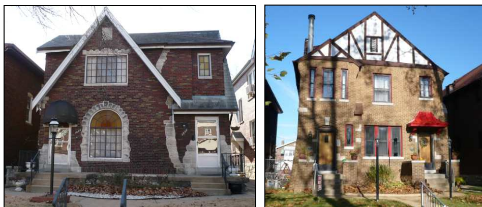
Figure 14: 3830 Fillmore (left) and 3945 Fillmore. Source: Holly Hills Survey, 2009.
