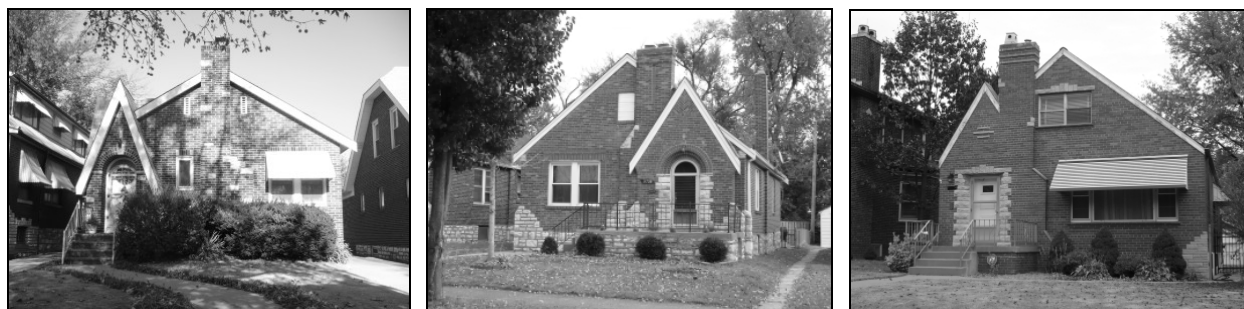
Figure 13: 3833 Dover (left; J. Myers, 1930); 5708 Arendes (no architect listed, 1939); and 3885 Federer Place (Bert Luer, 1955). Source: Holly Hills Survey, 2009. Source: Holly Hills survey, 2009.
