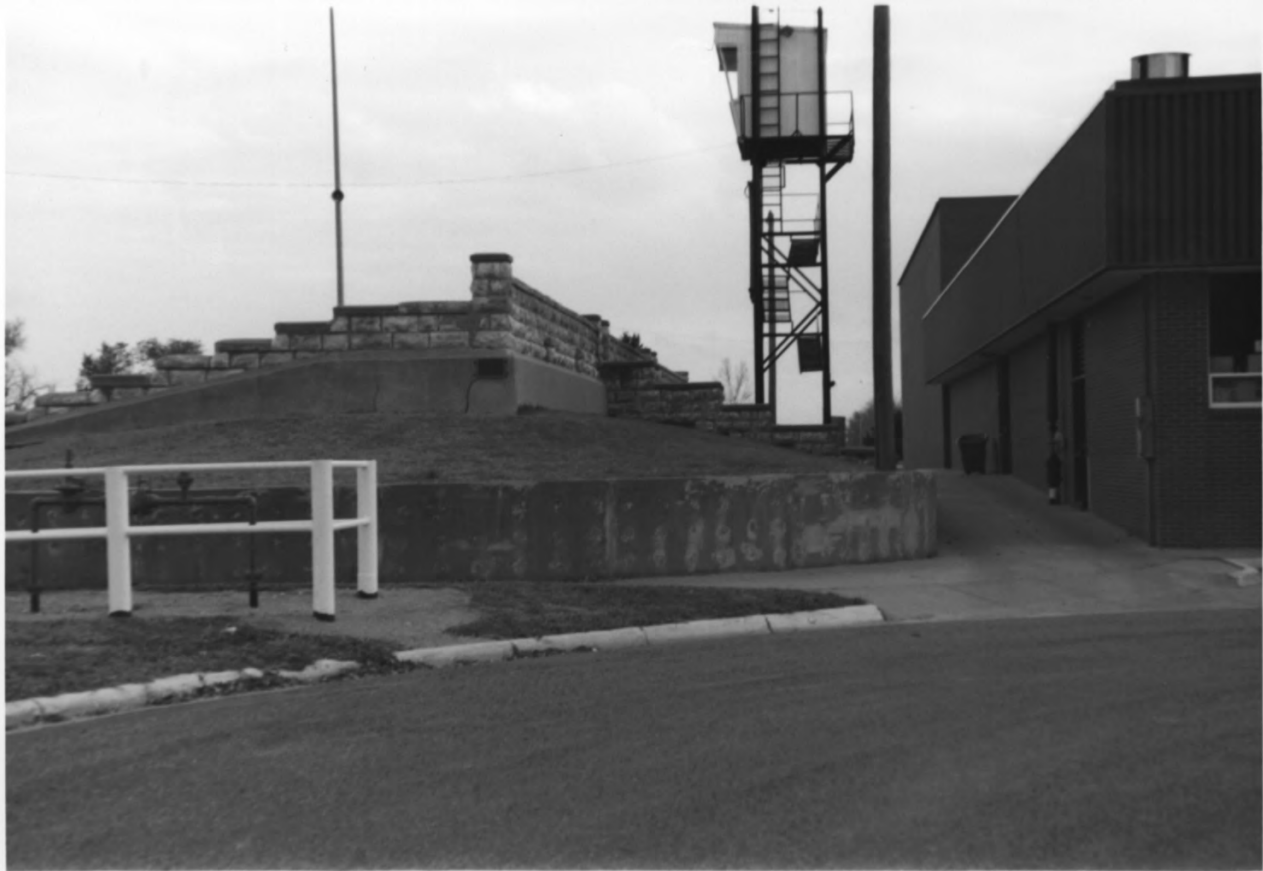
LANE COUNTY COMMUNITY HIGH SCHOOL, DIGHTON, KANSAS #8
