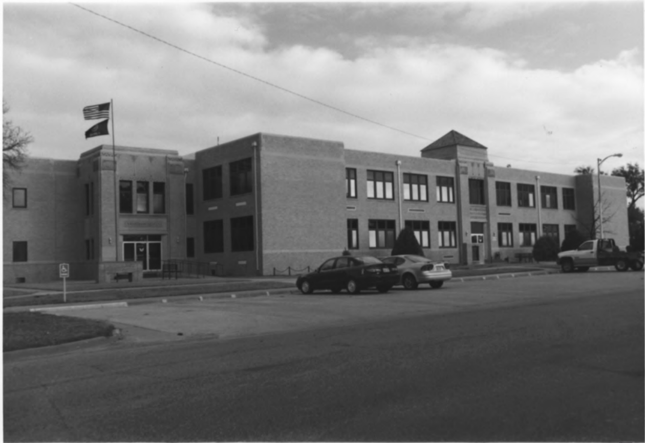
LANE COUNTY COMMUNITY HIGH SCHOOL, DIGHTON, KANSAS
