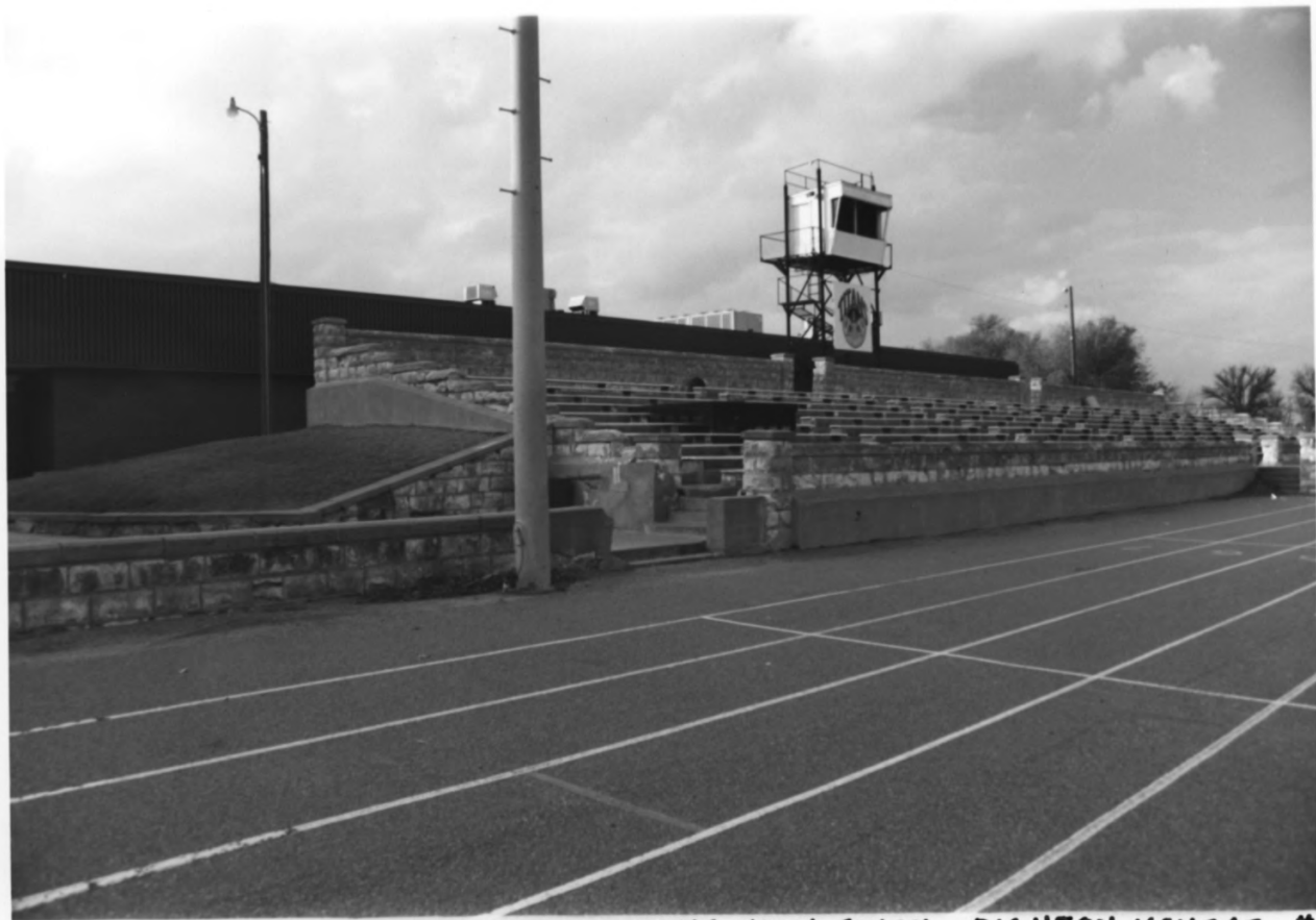
LANE COUNTY COMMUNITY HIGH SCHOOL, DIGHTON, KANSAS #7
