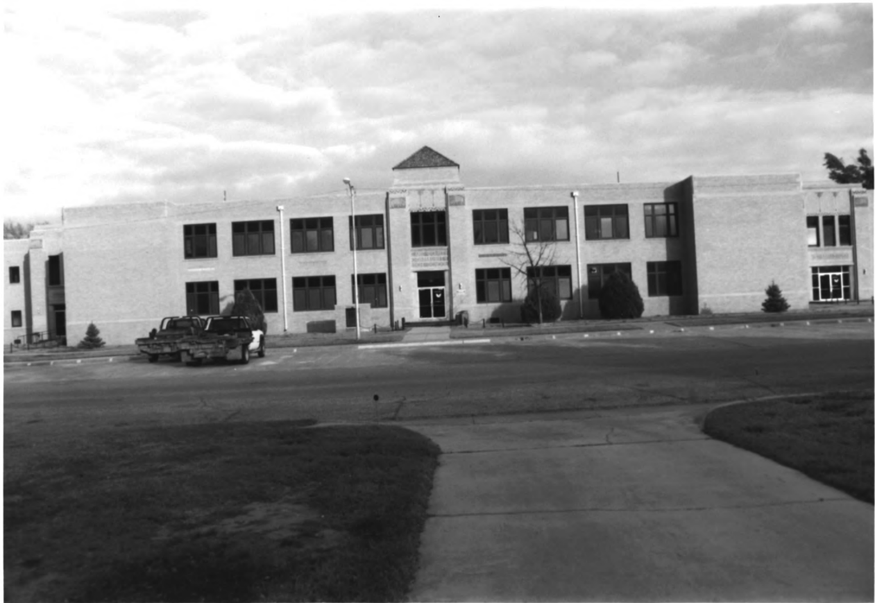
LANE COUNTY COMMUNITY HIGH SCHOOL, DIGHTON, KANSAS
