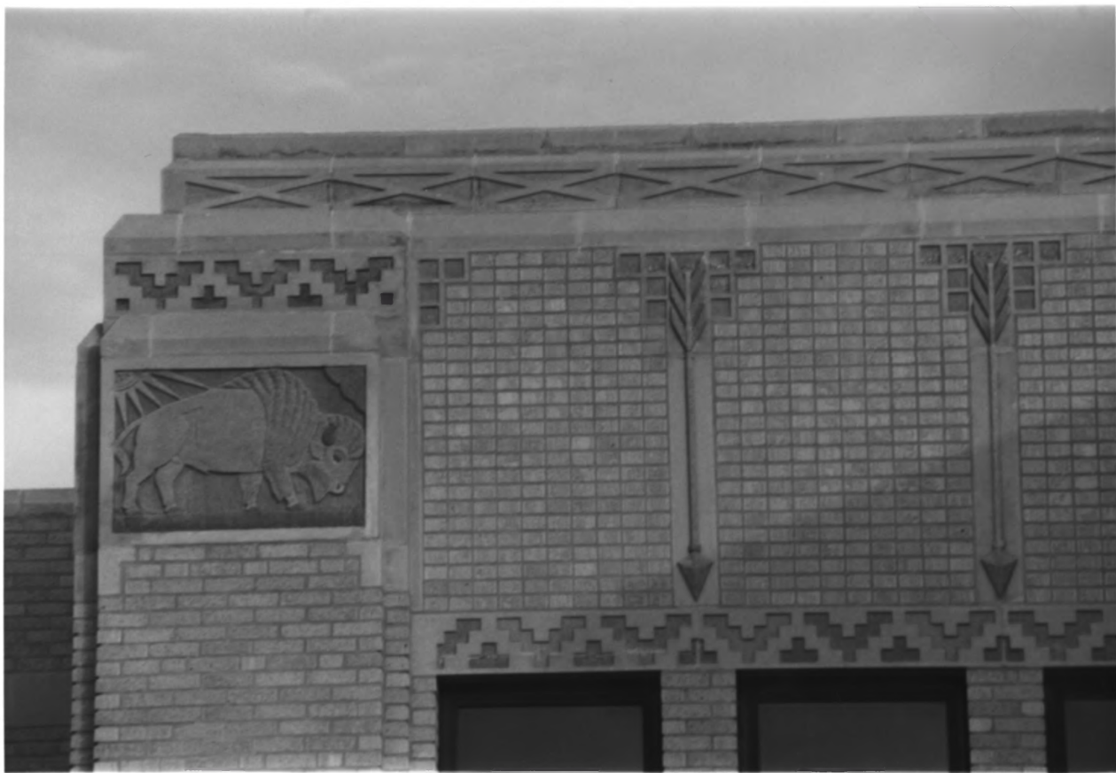
LANE COUNTY COMMUNITY HIGH SCHOOL, DIGHTON, KANSAS
