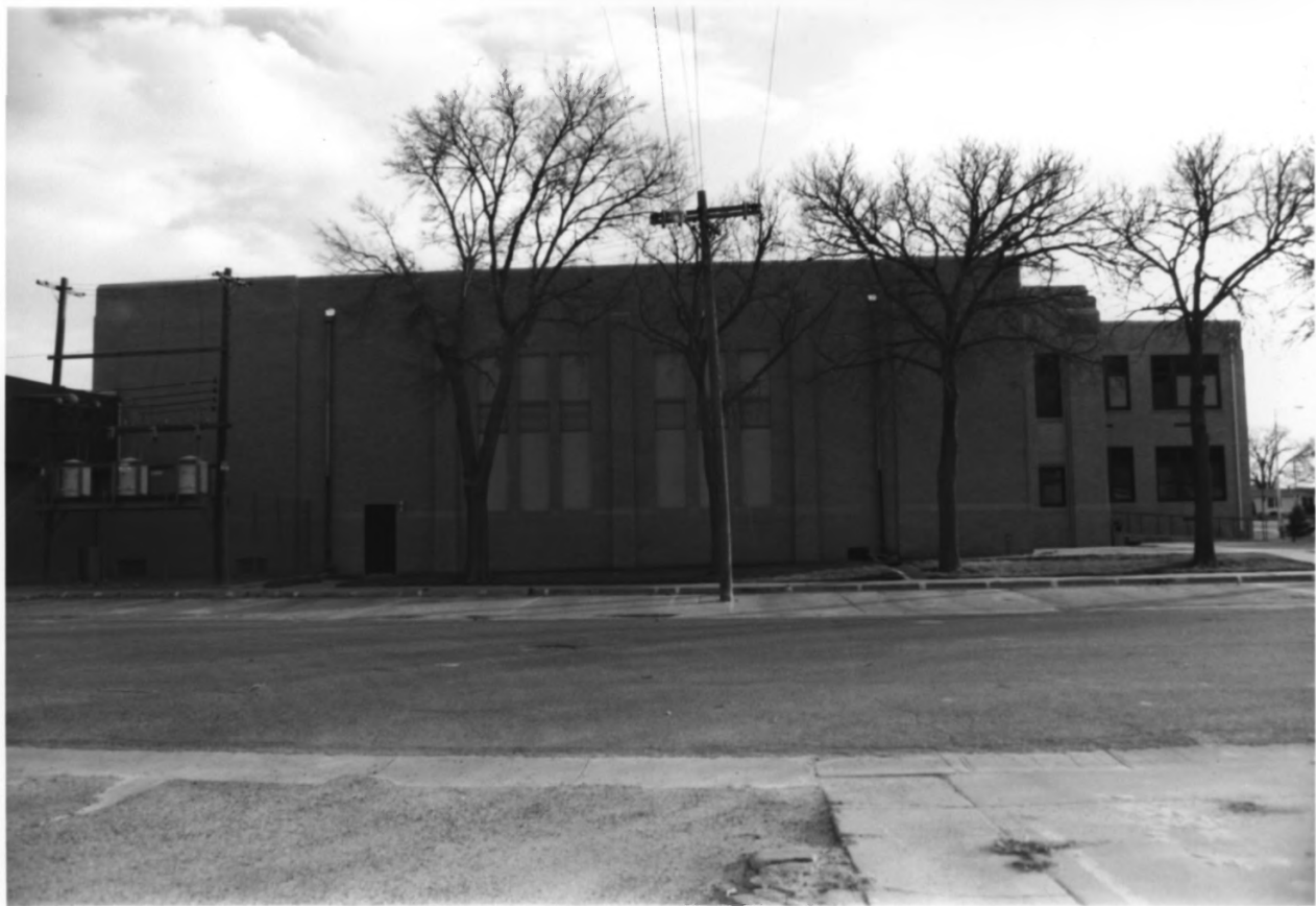
LANE COUNTY COMMUNITY HIGH SCHOOL. DIGHTON, KANSAS #10
