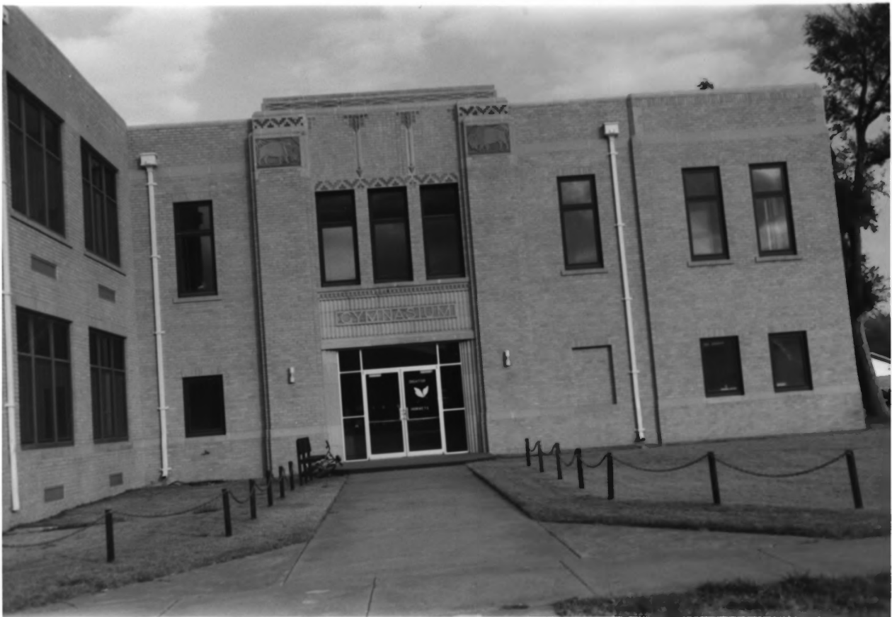
LANE COUNTY COMMUNITY HIGH SCHOOL, DIGHTON, KANSAS 45
