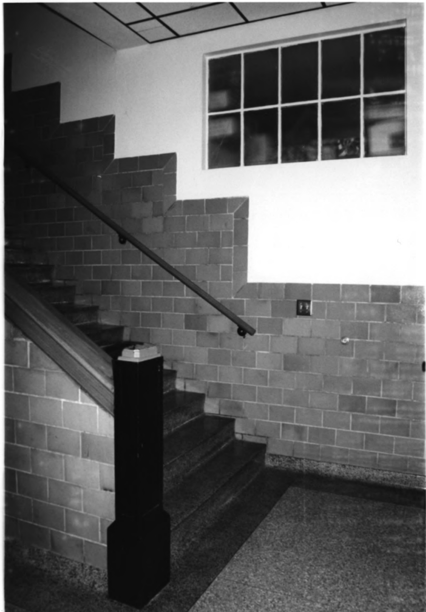
LANE COUNTY COMMUNITY HIGH SCHOOL, DIGHTON, KANSAS #14
