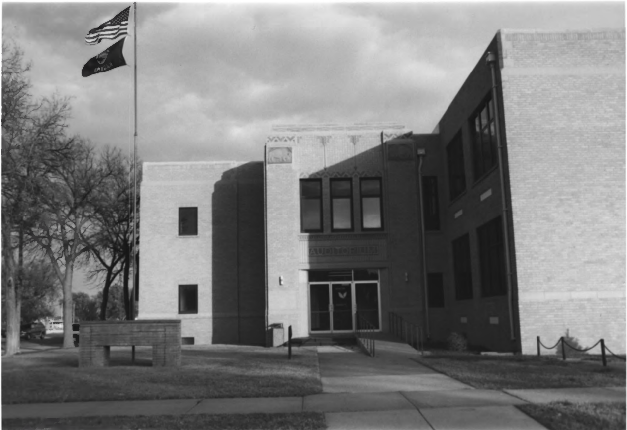
LANE COUNTY COMMUNITY HIGH SCHOOL, DIGHTON, KANSAS #11
