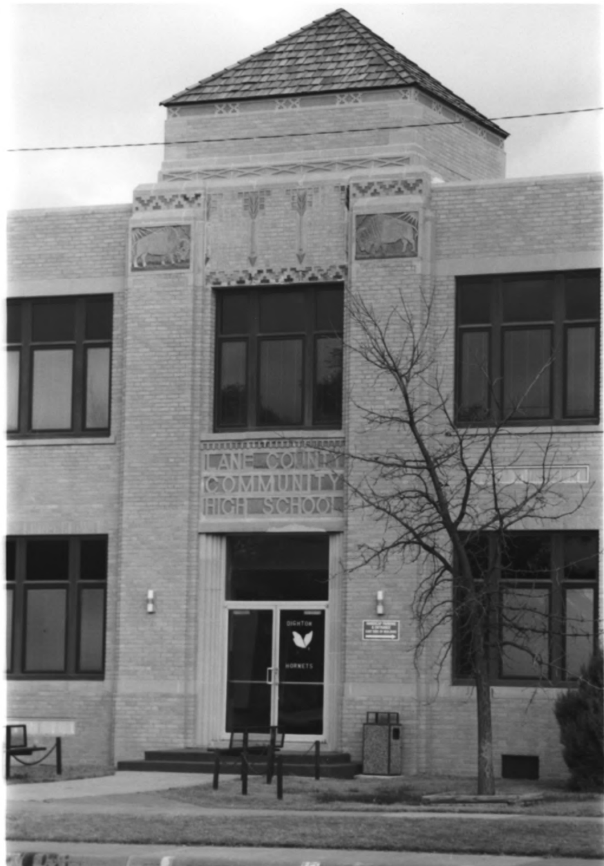
LANE COUNTY COMMUNITY HIGH SCHOOL, DIGHTON, KANSAS #2
