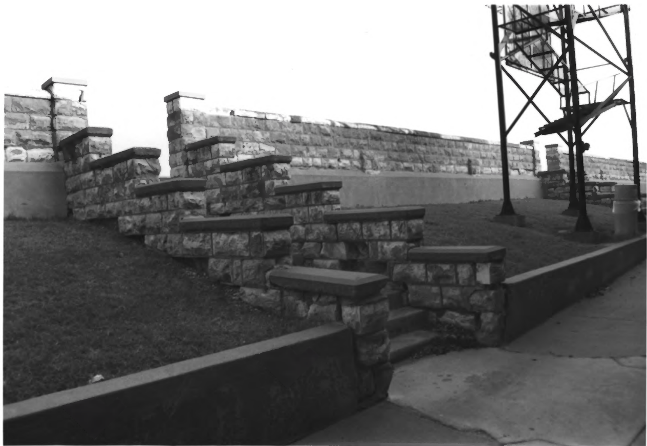
LANE COUNTY COMMUNITY HIGH SCHOOL, DIGHTON, KANSAS # 9
