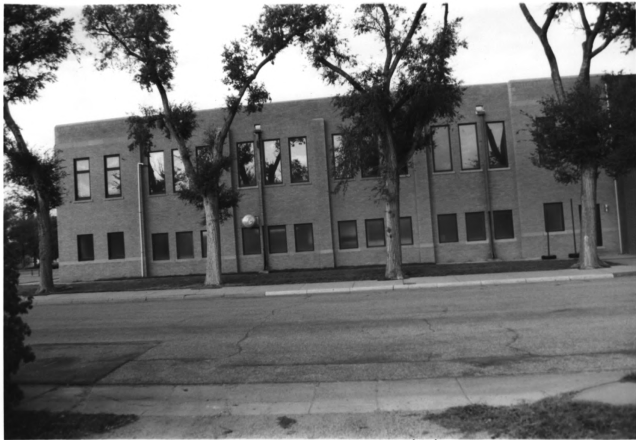
LANE COUNTY COMMUNITY HIGH SCHOOL, DIGHTON, KANSAS #6
