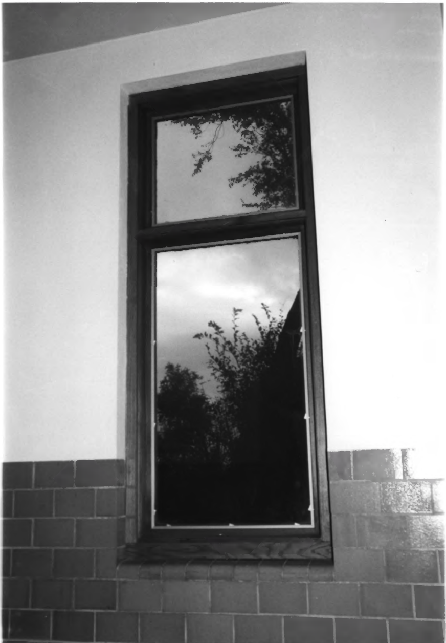
LANE COUNTY COMMUNITY HIGH SCHOOL, DIGHTON, KANSAS #16
