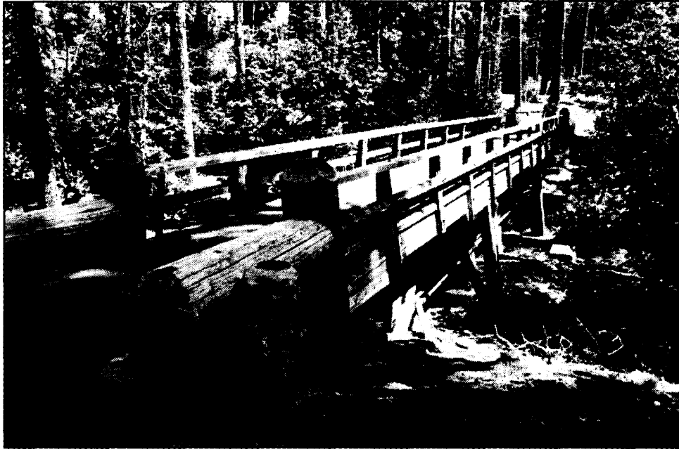
Photo 14: Bridge over Manzanita Creek.
