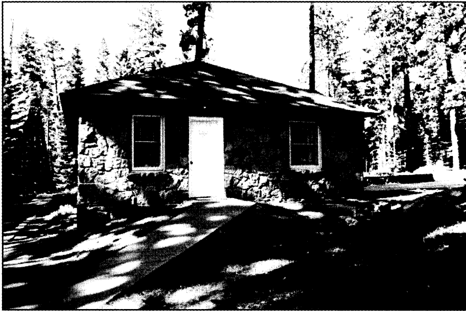
Photo 8: Loomis Residence and Studio, North Elevation.
