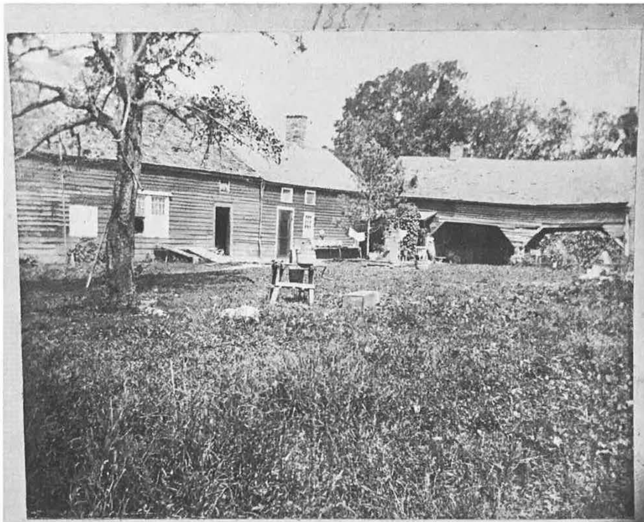
Figure 7: Historic photo (1889). East elevation (rear) of house looking west and north, showing clapboards, original cow shed
