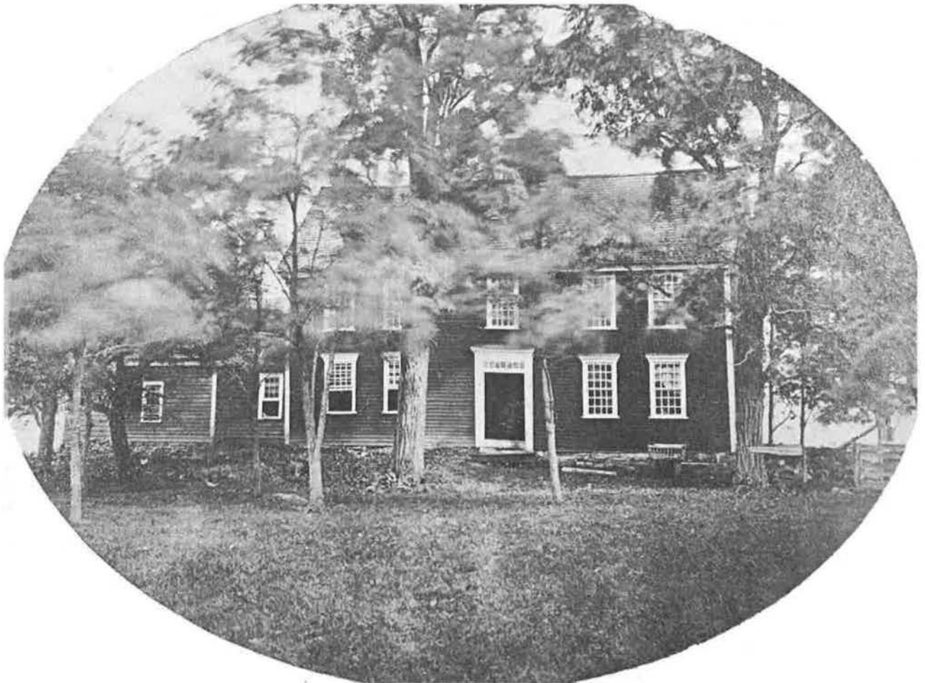
Figure 6: Historic Photo (undated). Front (west elevation) of house looking east. Earliest known picture of the house, shows clapboard, transom over front doors, no exterior porches; wing addition to north (left) does not have a door. Ward Family Collection, Sheffield Historical Society Photographs.
