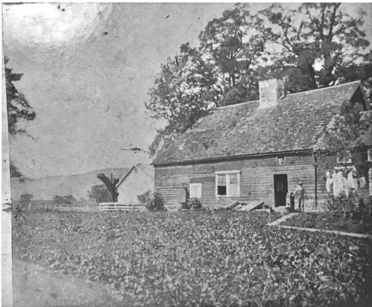
Figure 8: Historic photo (ca. 1889). East elevation (rear) of house looking southwest, probably same day as figure 7, shows barn to south (not extant).
