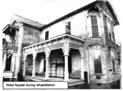
During the 2003-2005 rehabilitation, it was discovered that the original design may have included turned balusters and a railing on top of the porch roofs. Notches that matched the existing ground level porch railing shape and cut at the height of the existing ground level railings were found on the exterior walls by the roofs. Also, raised platforms that would have held a bottom railing were found on the porte cochere roof.
