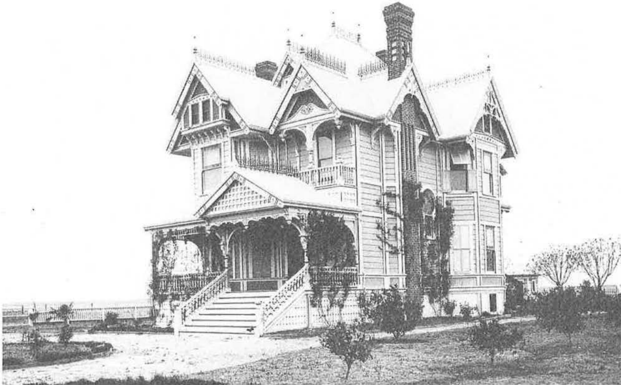
Figure 1: Historical photograph of the Bald Eagle Ranch House taken sometime after construction in 1893.
