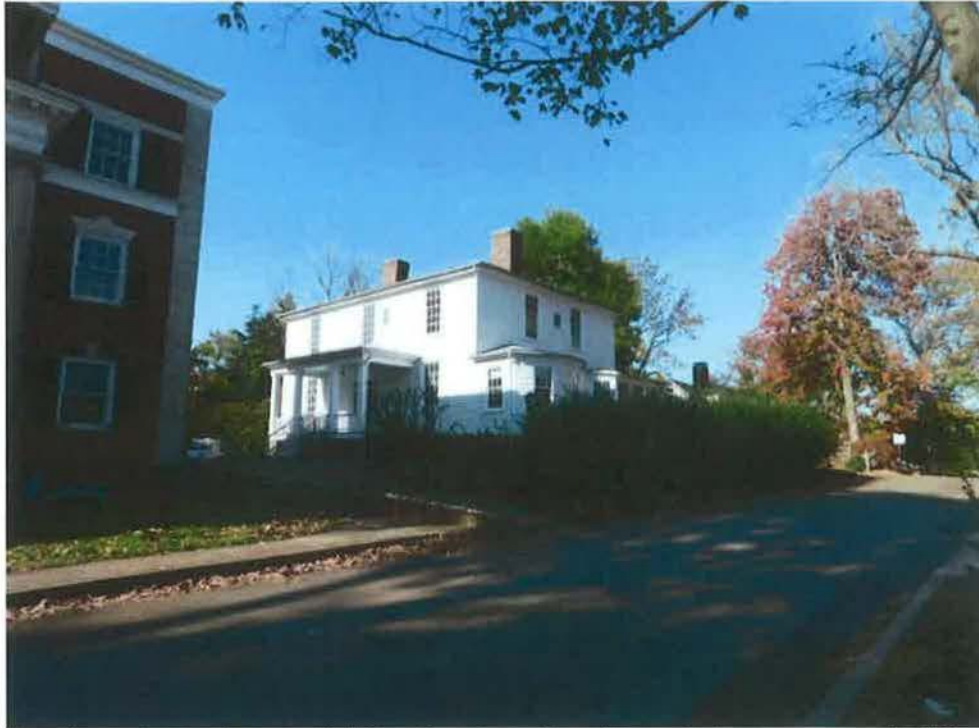
Current location of Wyndhurst, with façade oriented to the south (an apartment building, at left, is in the property's former front yard), camera facing north/northwest.
