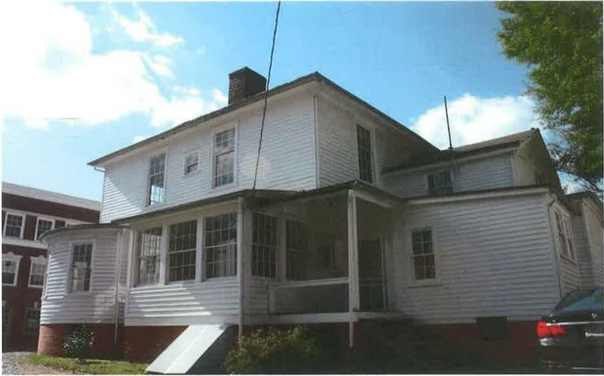
East Elevation (l), rear additions (r), view SW
