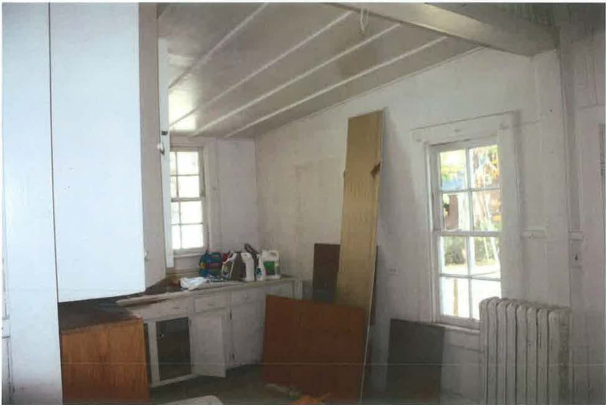
First Floor, rear NE addition to addition, view NE
