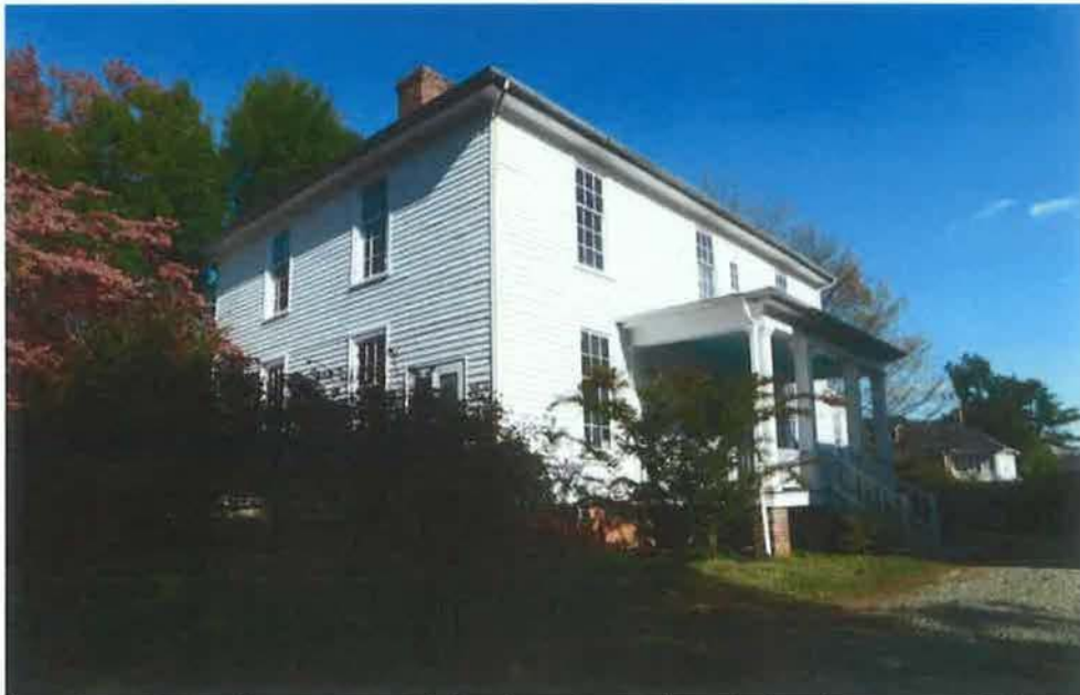
Current location of Wyndhurst, west (side) elevation and south façade, camera facing northeast.
