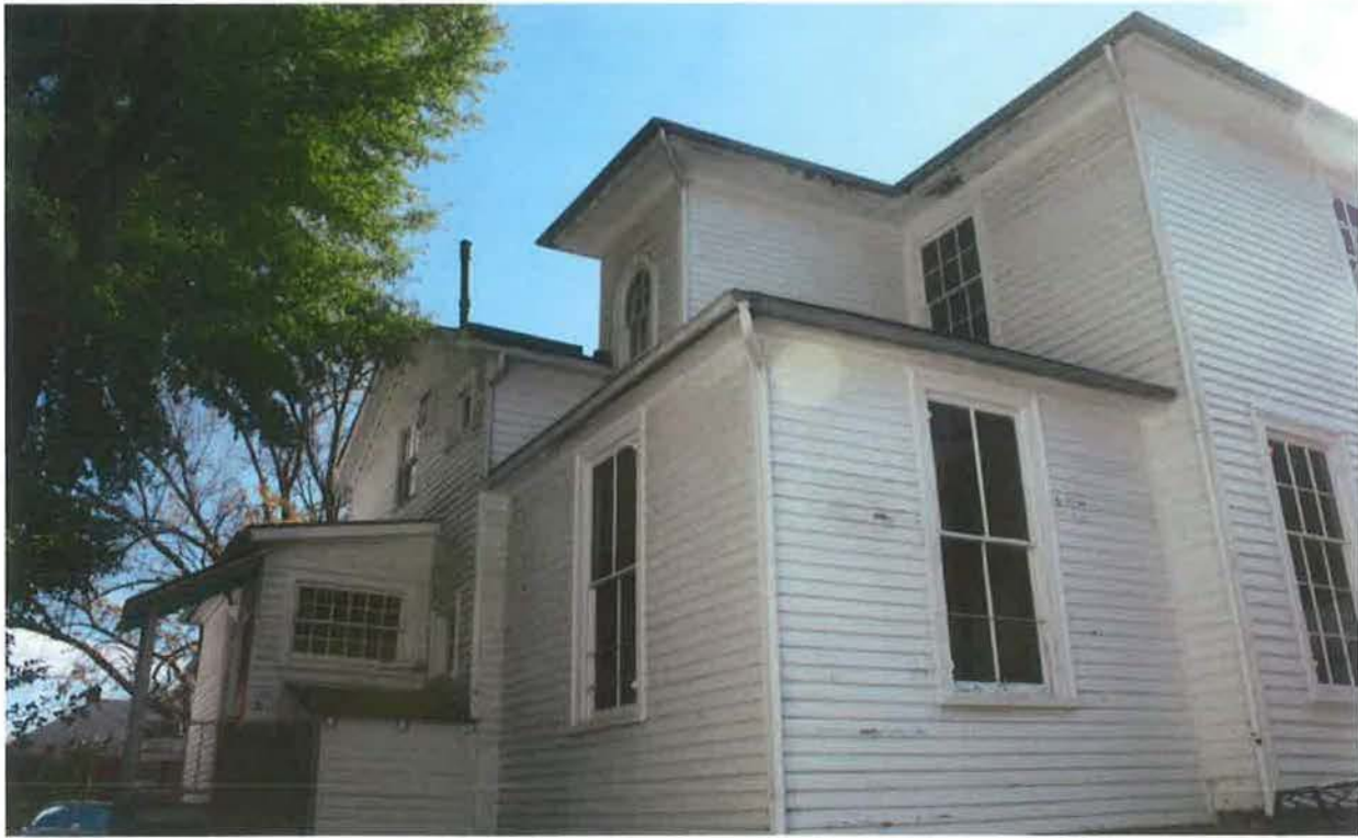
North (rear) elevation, view SE
