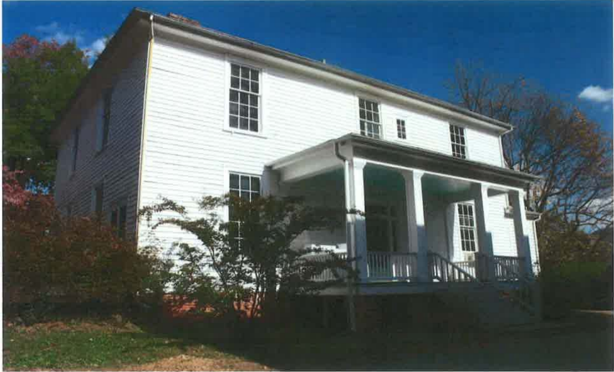
South Elevation, view NE
