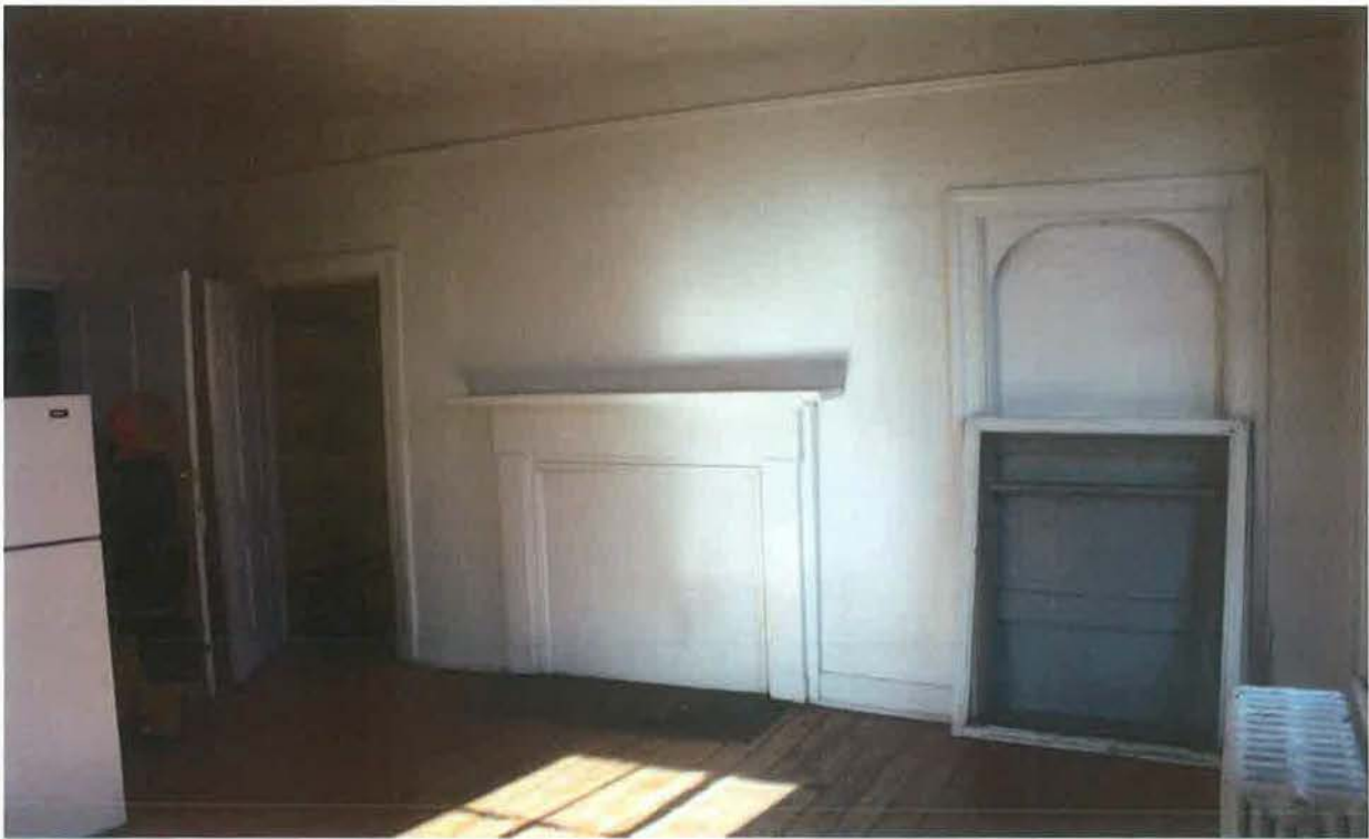
Second Floor, SE room, view NW
