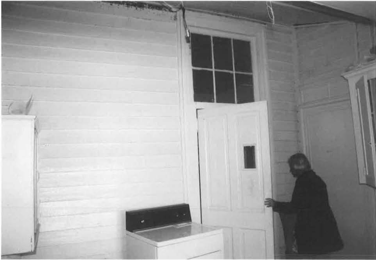
First Floor, rear NE addition adjoining main house, view SW
