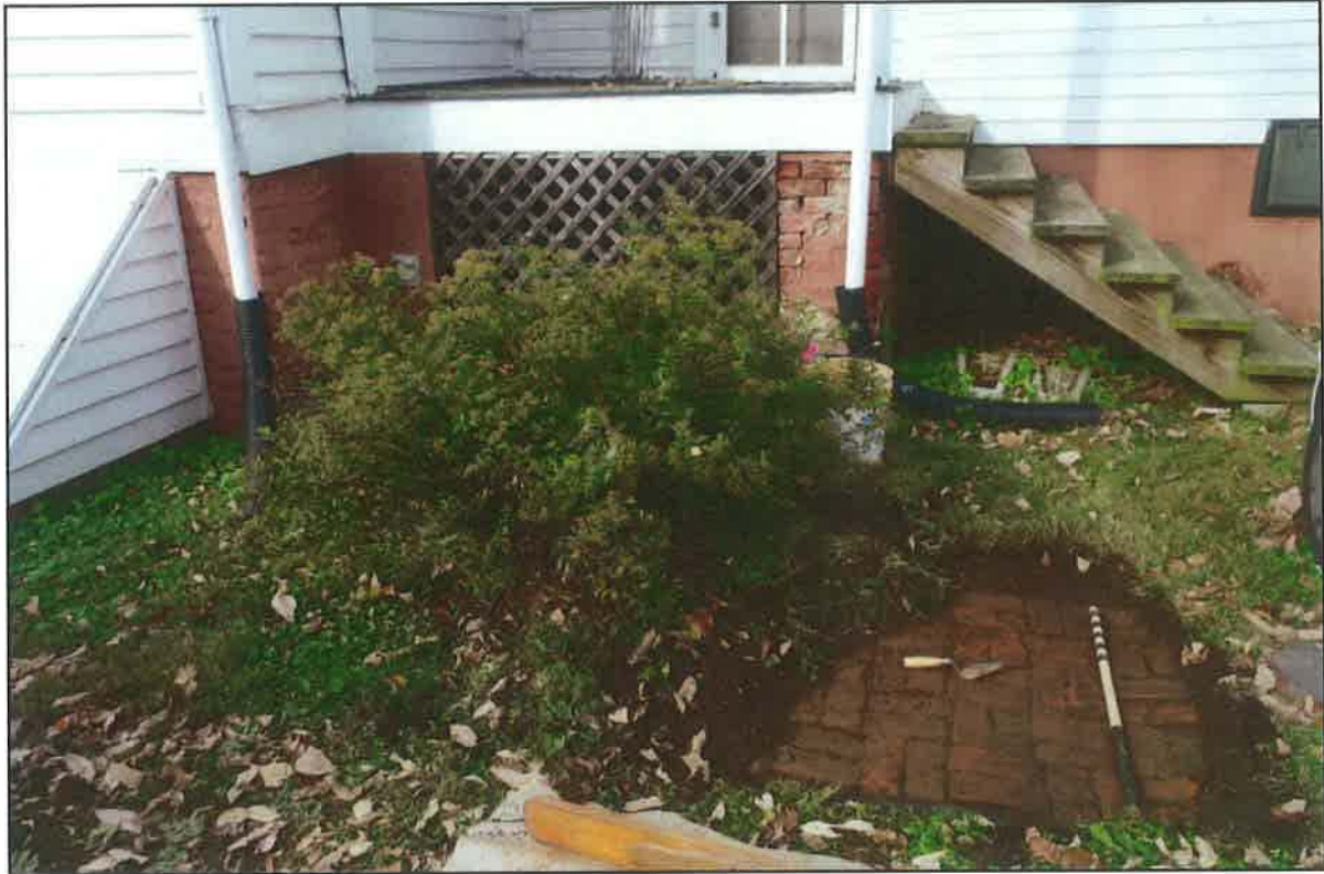
Figure 20: View facing west of the section of brick-paved walk exposed off the northeast corner of Wyndhurst.
