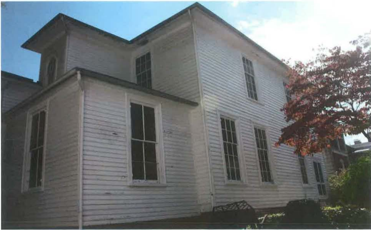
North (l) and West (r) elevations, view SE
