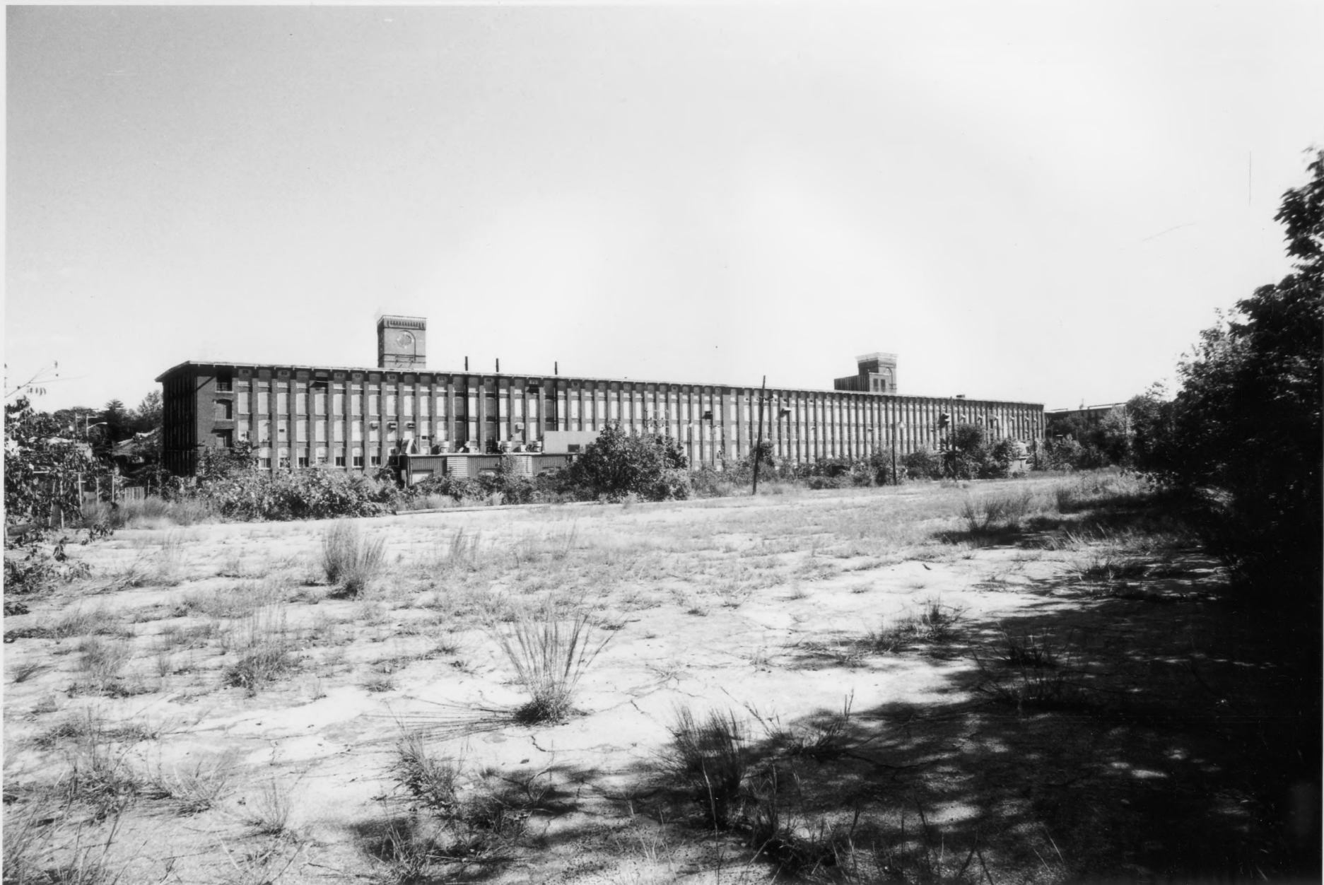
WEST ELEVATION OF MAIN MILL GREYSTONE MILL HISTORIC DISTRICT NORTH PROVIDENCE, PROVIDENCE COUNTY PHOTOGRAPH NUMBER 1 RHODE ISLAND
