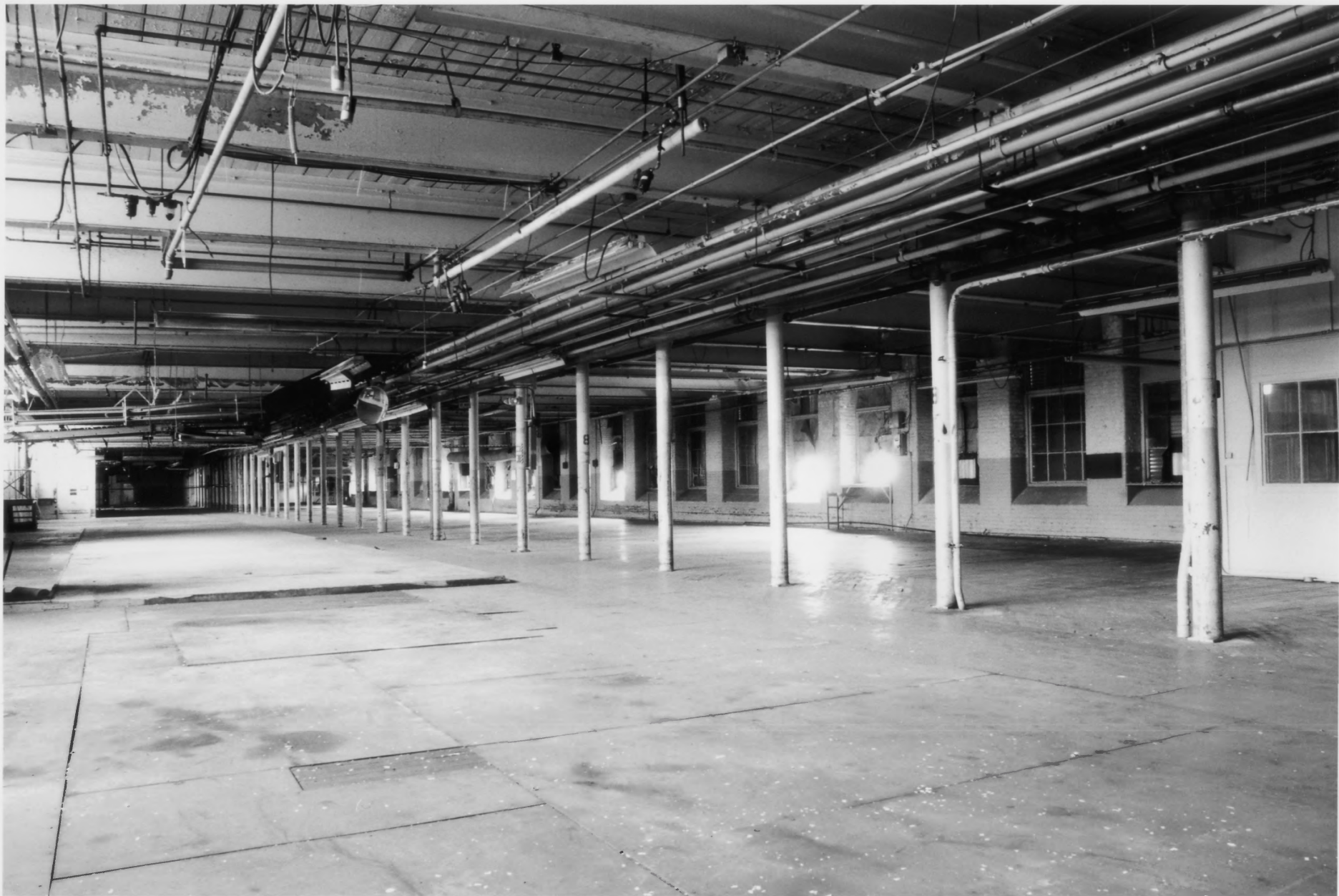
INTERIOR VIEW OF MAIN MILL GREYSTONE MILL HISTORIC DISTRICT NORTH PROVIDENCE, PROVIDENCE COUNTY RHODE ISLAND PHOTOGRAPH NUMBER 14
