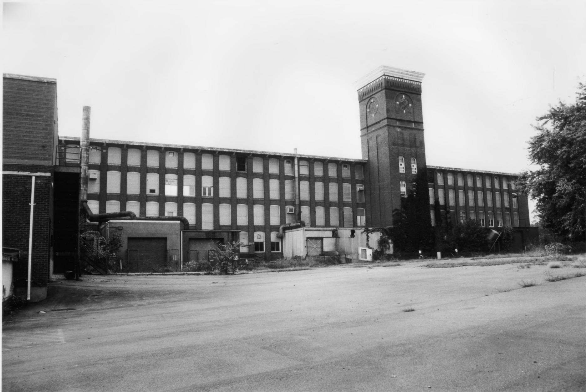
Main Mill and North Tower GREYSTONE Mill Historic District North Providence, Providence County Rhode Island Photograph Number 4
