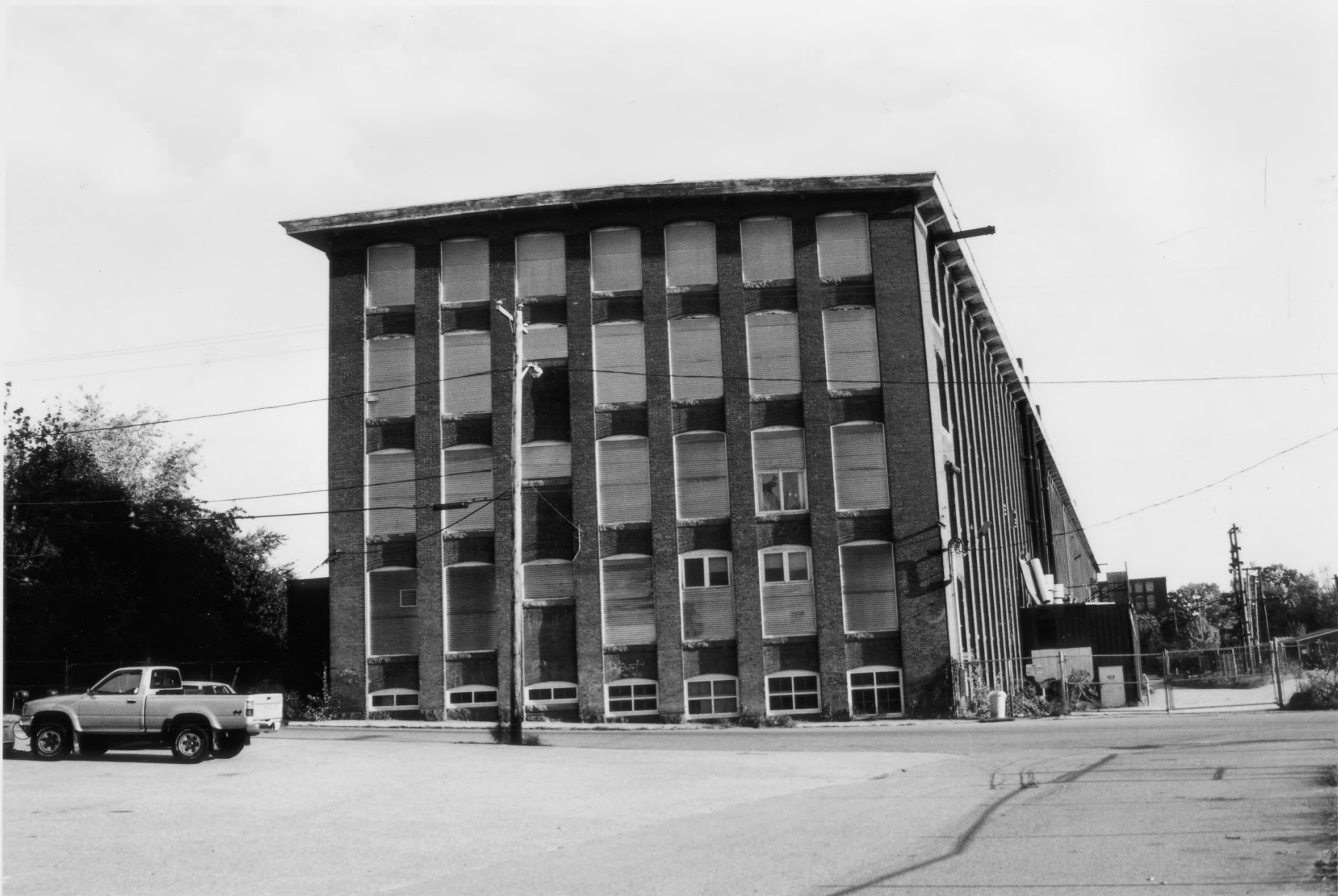
NORTH ELEVATION OF MAIN MILL GRAYSTONE MILL HISTORIC DISTRICT NORTH PROVIDENCE, PROVIDENCE COUNTY, RHODE ISLAND PHOTOGRAPH NUMBER 2
