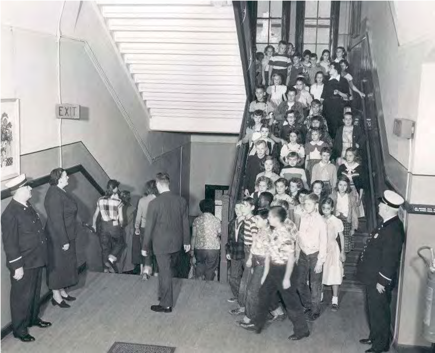
Figure 3: View of the west stairway during a fire drill, 1953. Chuckman Collection.
