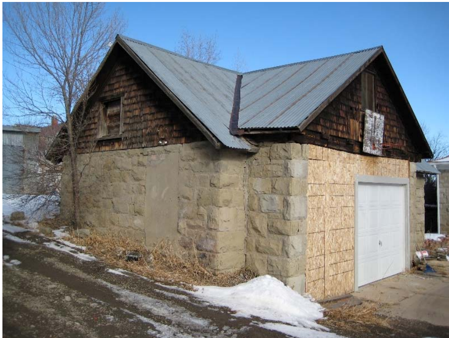
Fig 17 - West and south side of garage. Camera pointing northeast. Photo by Fritz Augustin, 2008.
