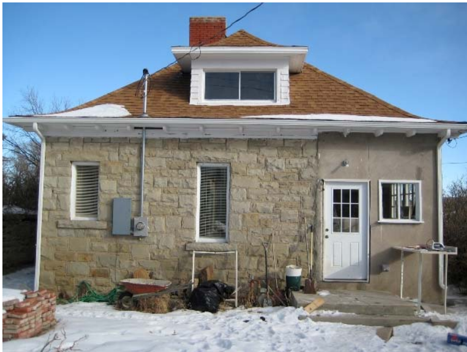
Fig 15 - West side of house. Camera pointing east. Photo by Fritz Augustin, 2008.
