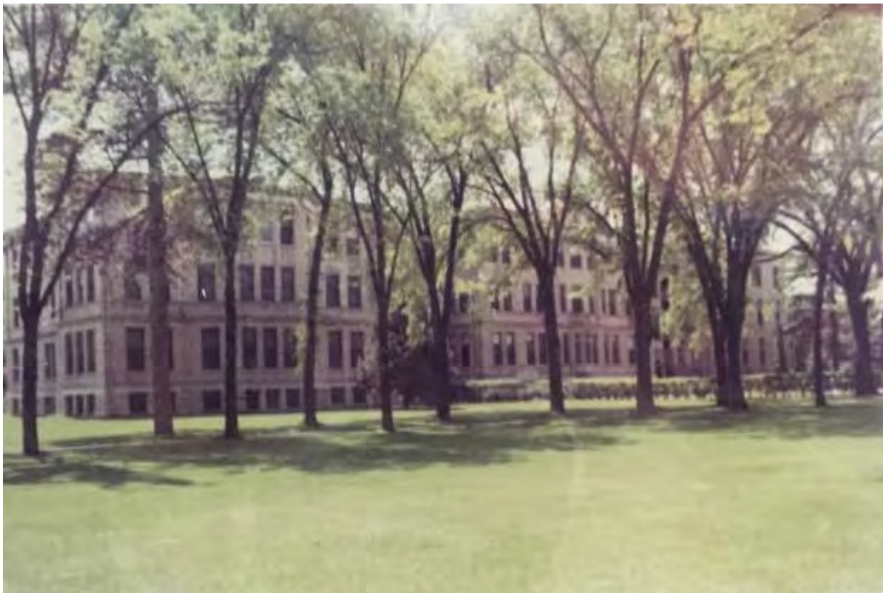
Figure 15: May 1969 photograph looking southwest toward the north facade.
