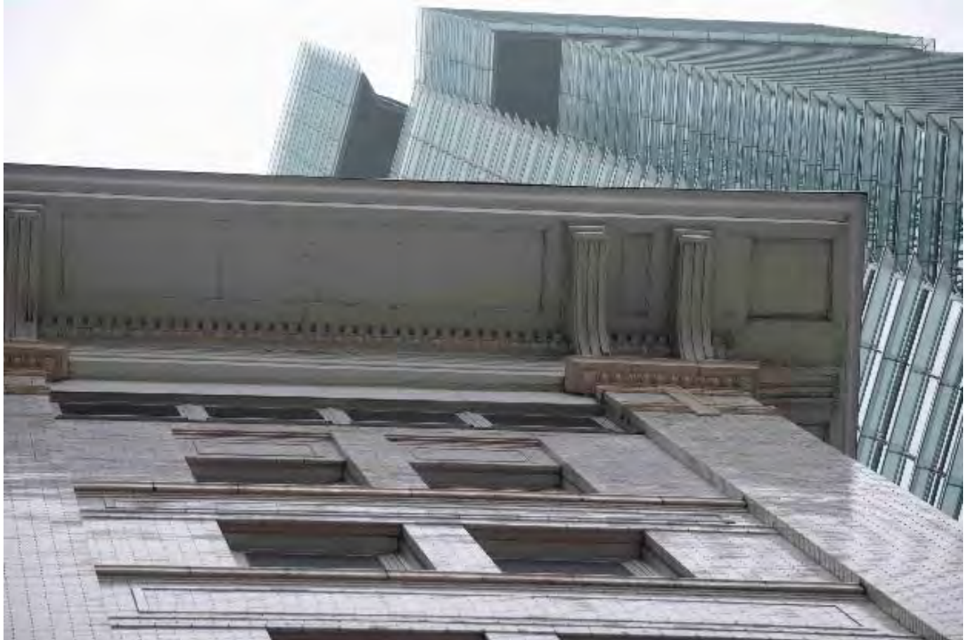
Photo #5 East elevation, detail of cornice and glazed brick, 2014.
