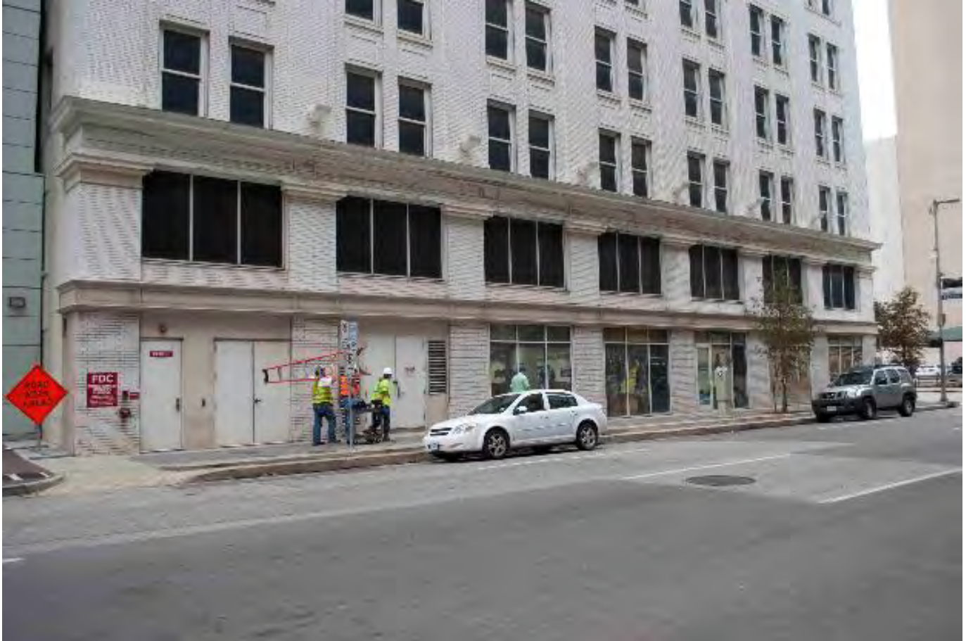
Photo #11 South elevation, detail of ground floor storefront, camera facing northeast, 2014.
