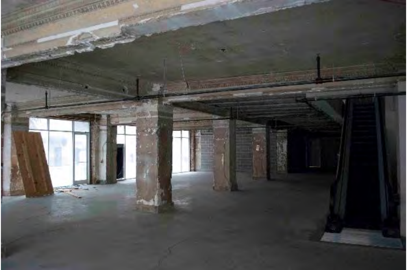
Photo #6 Interior, tenth floor, camera facing south, 2014.
