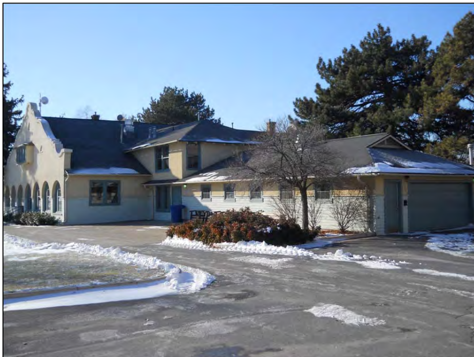
Photograph 8. Overview of clubhouse (2015); looking southwest
