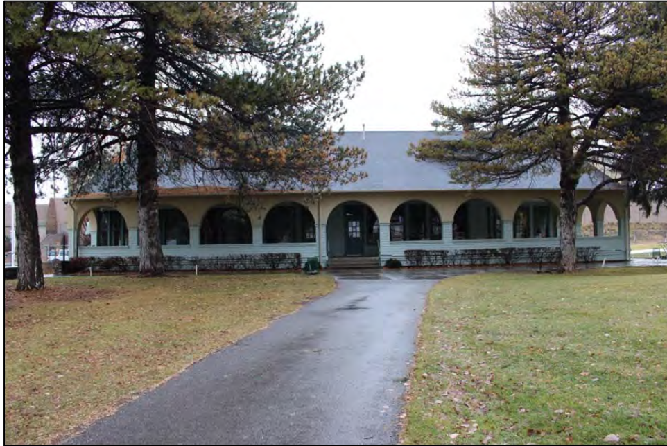
Photograph 11. South elevation of clubhouse (2015); looking north
