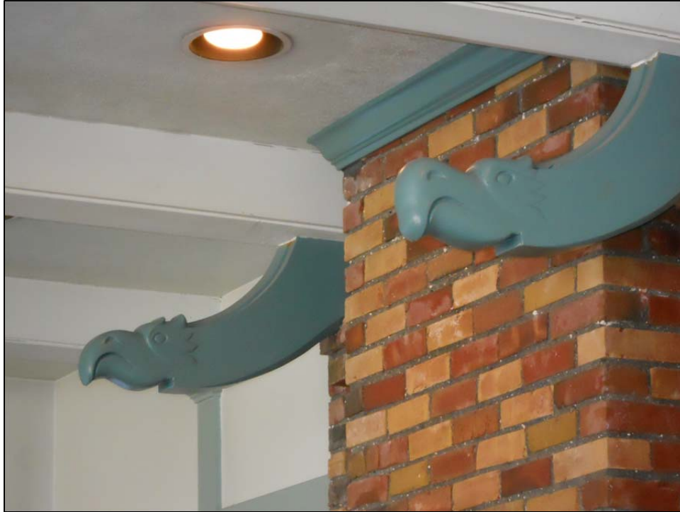
Photograph 20. Example of historical interior finishes and detail (2015); close-up
