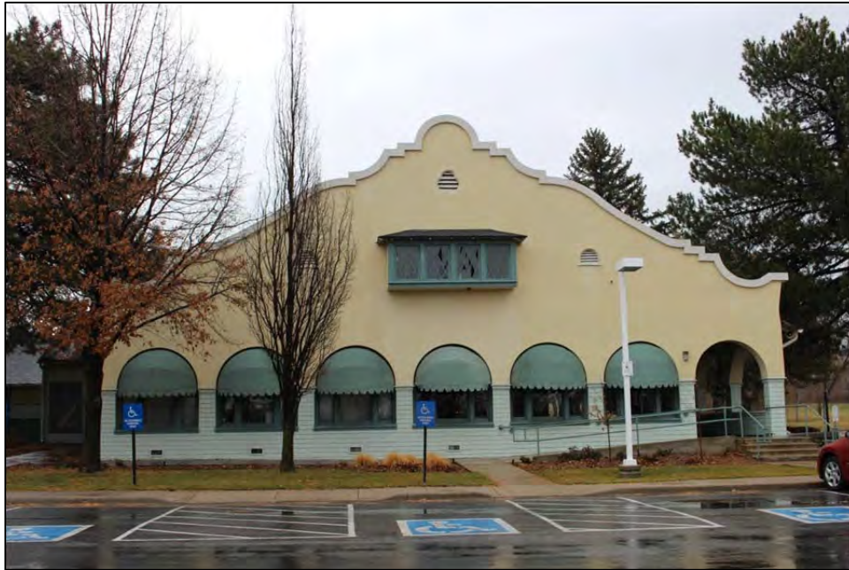
Photograph 9. West elevation of clubhouse primary volume (2015); looking east
