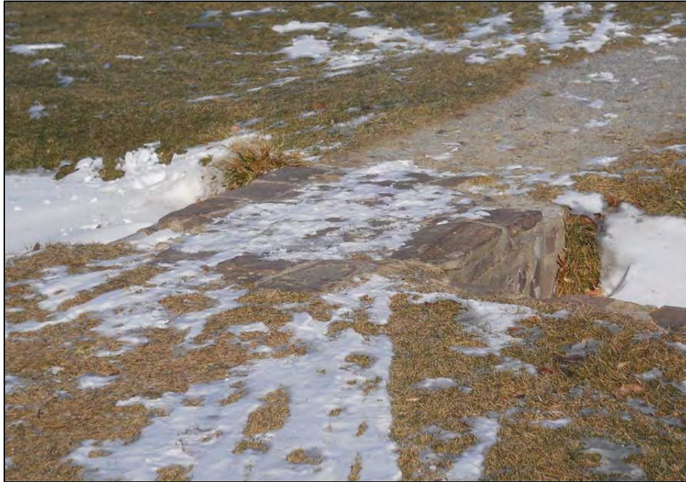
Photograph 22. Example of non-contributing stone culvert (2015); looking northeast
