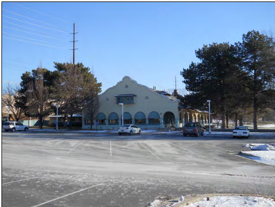
Photograph 6. General overview of clubhouse (2015); looking east-northeast
