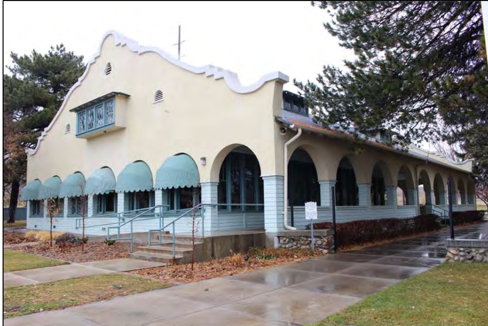
Photograph 17. West and south elevations of clubhouse (2015); note veranda along south elevation; looking northeast
