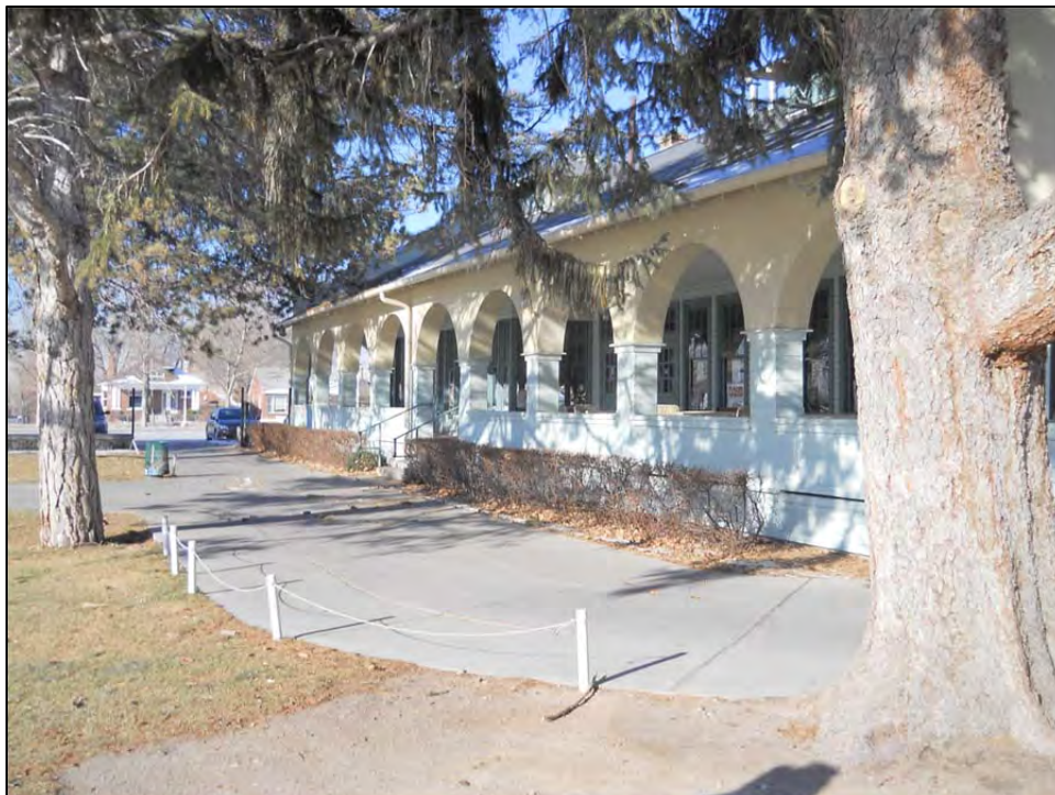
Photograph 18. South elevation of clubhouse showing veranda (2015); looking northwest
