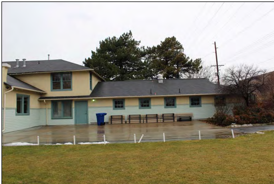
Photograph 14. East elevation of clubhouse northern ell and garage addition (2015); looking west
