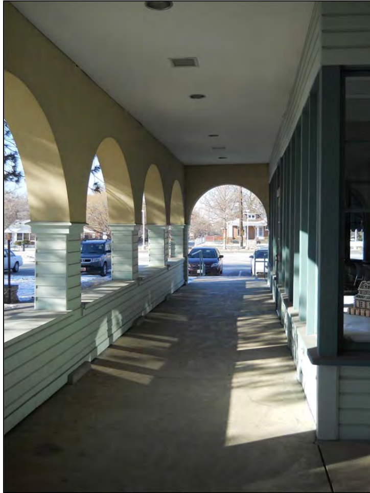
Photograph 19. Interior of southern veranda (2015); looking west clubhouse (2015); looking west
