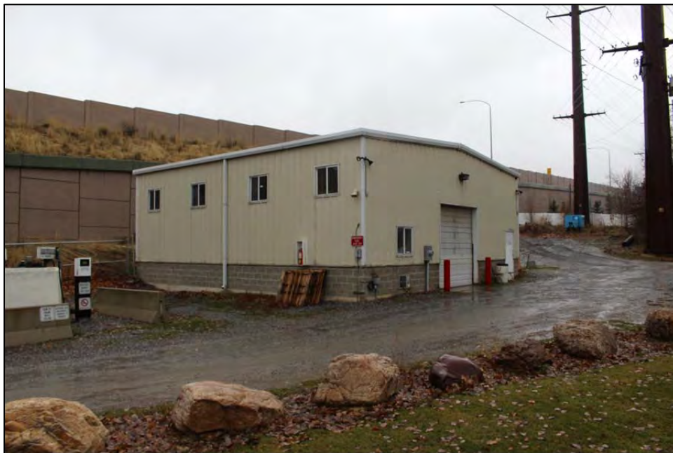
Photograph 21. Non-contributing maintenance shed—Building 1 (2015); looking northeast
