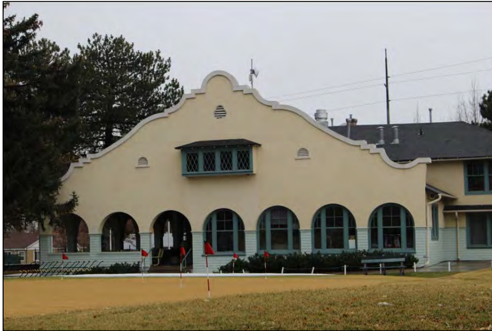
Photograph 13. East elevation of clubhouse primary volume (2015); looking west
