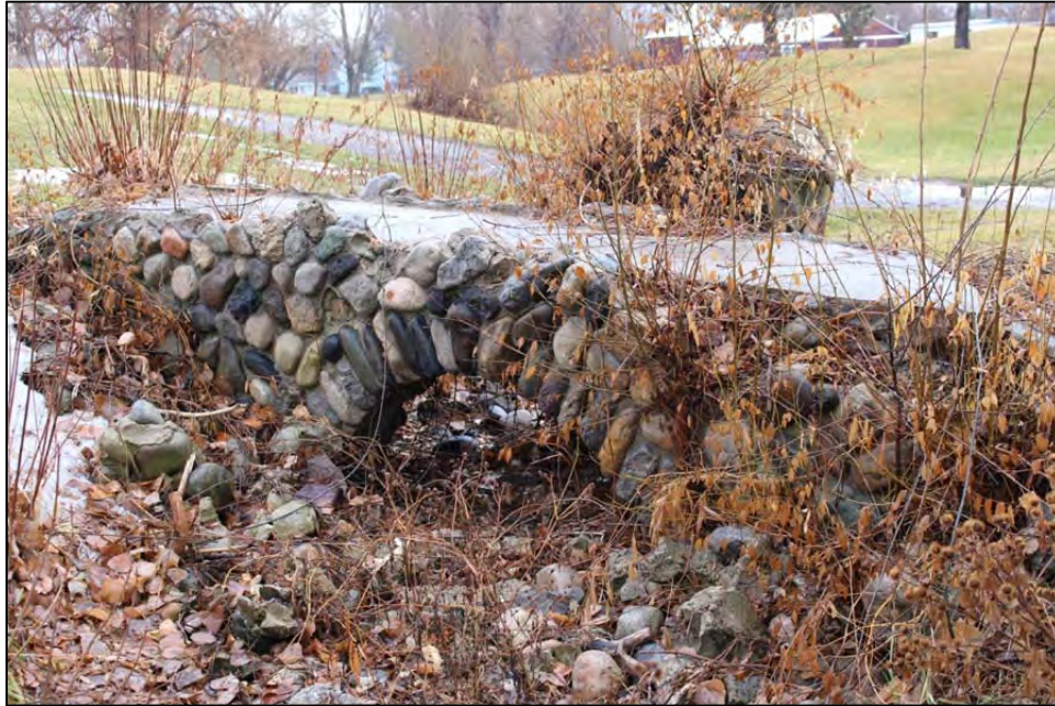
Photograph 5. Stone bridge (2015); looking northeast
