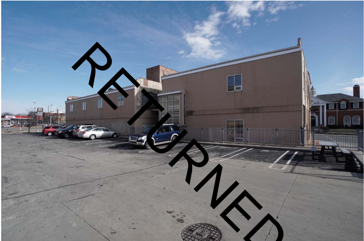
Figure 27: West façade; view facing northeast (Photo 3).
