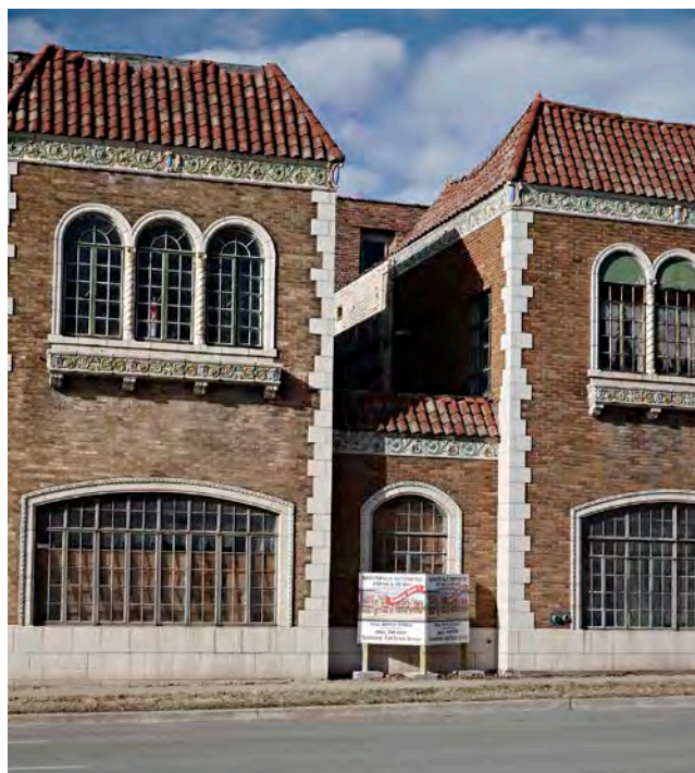
Figure 10: Details of terra cotta elements featured on the east façade of the south unit (above).
