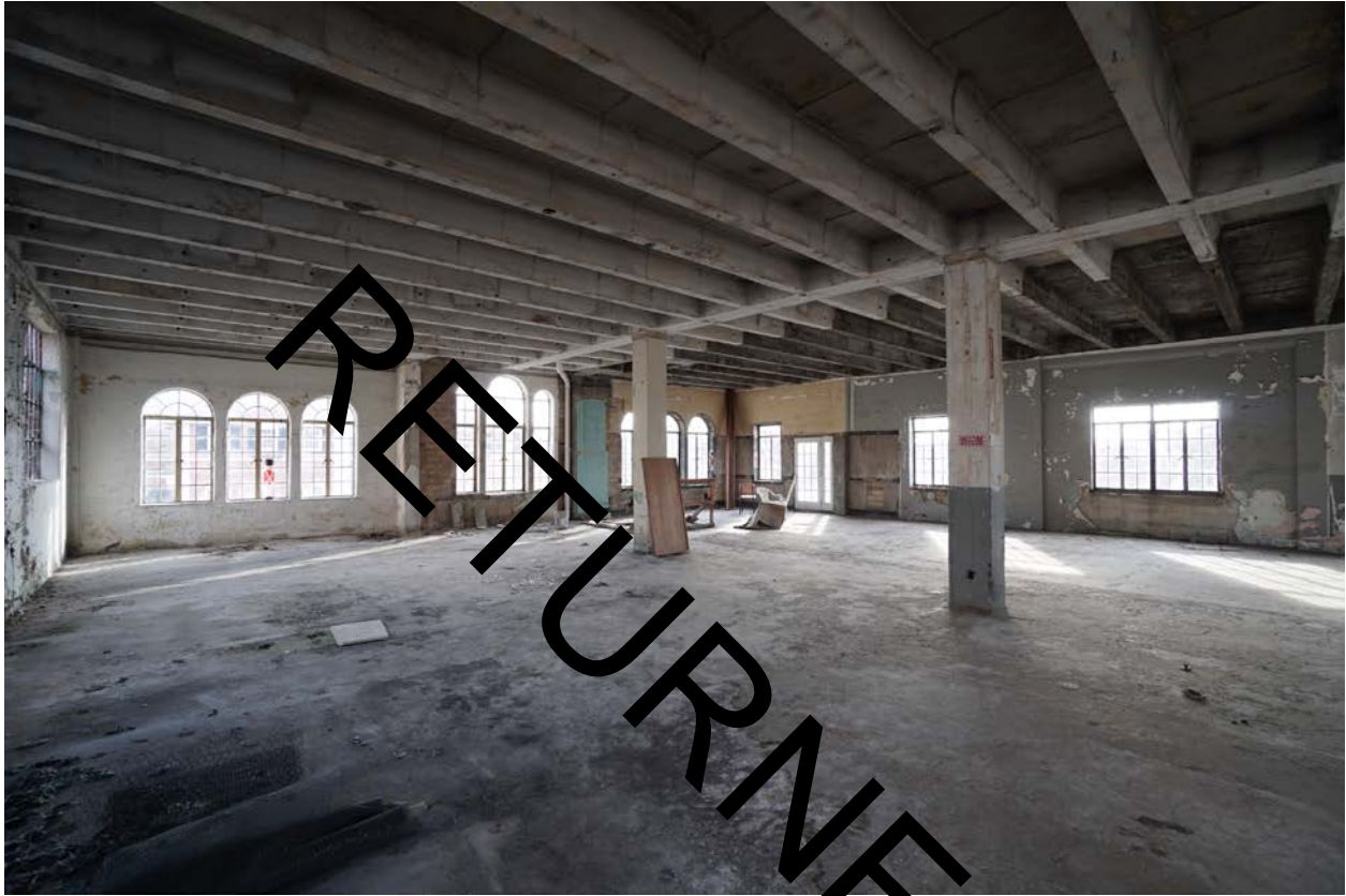
Figure 31: South unit interior, second floor; view facing southeast (Photo 7).
