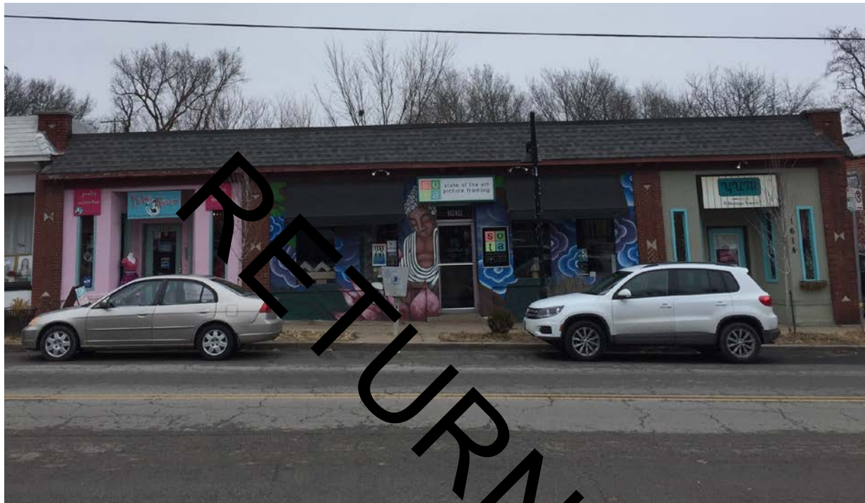
Figure 22: 4112-14 Troost Avenue (above) and 1414-24 W 39 th Street (below).
