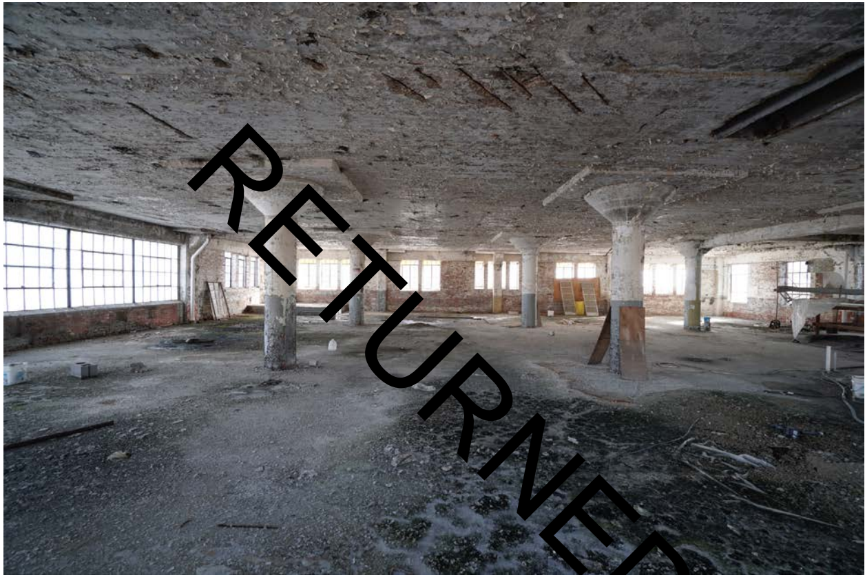
Figure 33: North unit interior, second floor; view facing east (Photo 9).
