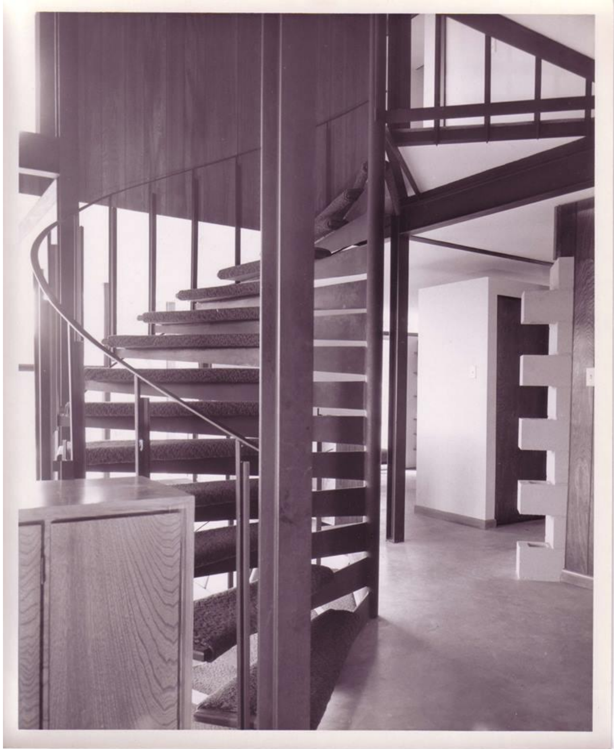
Figure 7: Historic photo of the staircase of the Wanslow House, looking southwest, c.1962.
