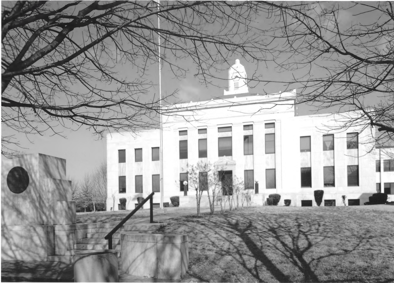
HALL COUNTY COURTHOUSE HALL COUNTY, GEORGIA 1 OF 7
