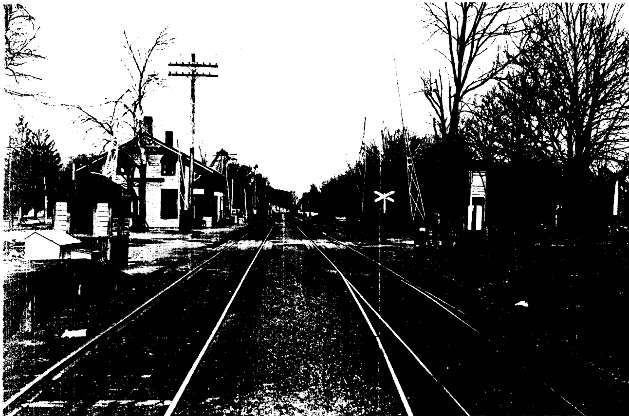
second track was added at Morris Plains in 1902-3, but it was not until 1915 that the community received a new station. This view was taken in February 1915 looking west, just prior to the start of the grade separating work.
