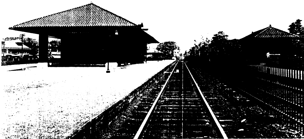
The tracks at Morris Plains were elevated several feet. There was sufficient room for the roads to be depressed under the tracks. As with Convent, Morris Plains also received a small freight house which in this photo has a box car spotted near it. This view looks west.
