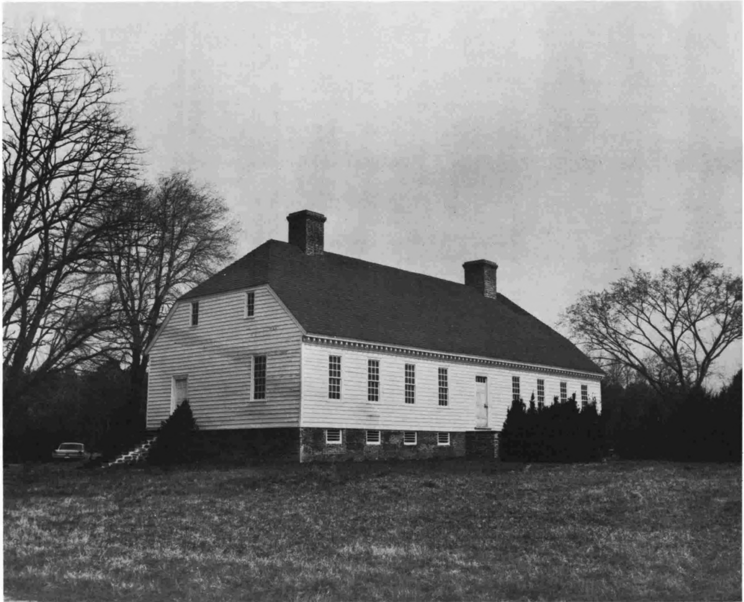
Scotchtown - gable end
