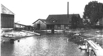
Ca. early 1900s historic photograph of the sawmill and mill pond formerly located within the Covenant Beach Bible Camp valley. Source: Digital copy provided by Carmen Scott.
