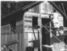
ca. 1909 construction of one of the Women's Lark Cabins. Source: Digital copy provided by Carmen Scott.
