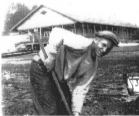
1923 photograph of the former Church Hall with Bob Bernick, a former camp attendee, in the foreground. Source: Digital copy provided by Carmen Scott.
