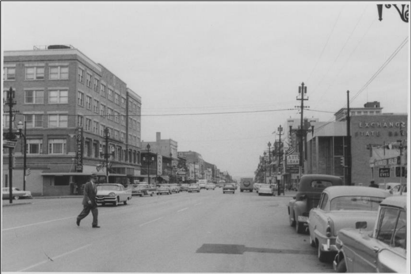
Figure 9. Minnesota Avenue, looking east in 1957. Old Brotherhood Building is at left and shows building's cornice has been removed and a new flat awning installed at first floor [Source: Kansas Memory, State Archives, Kansas Historical Society].
