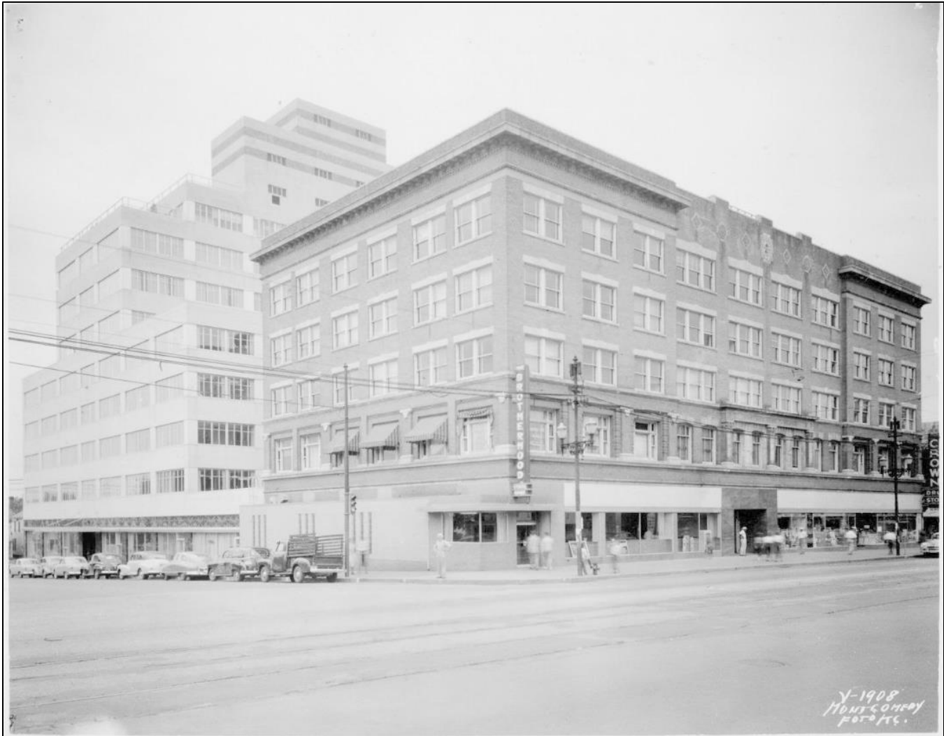
Figure 8. Brotherhood Block, view NE from the intersection of Eighth & Minnesota. 1951. Notice cornice of Old Brotherhood Building is in place and street level has been altered. [Source: Missouri Valley Special Collections, Kansas City (Missouri) Public Library]
