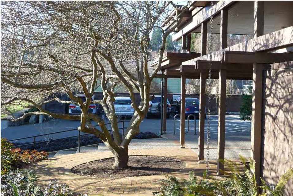
Photo #4 Exterior view of landscaping at main entry, camera facing west Photographer: Susan Boyle, January 14, 2015
