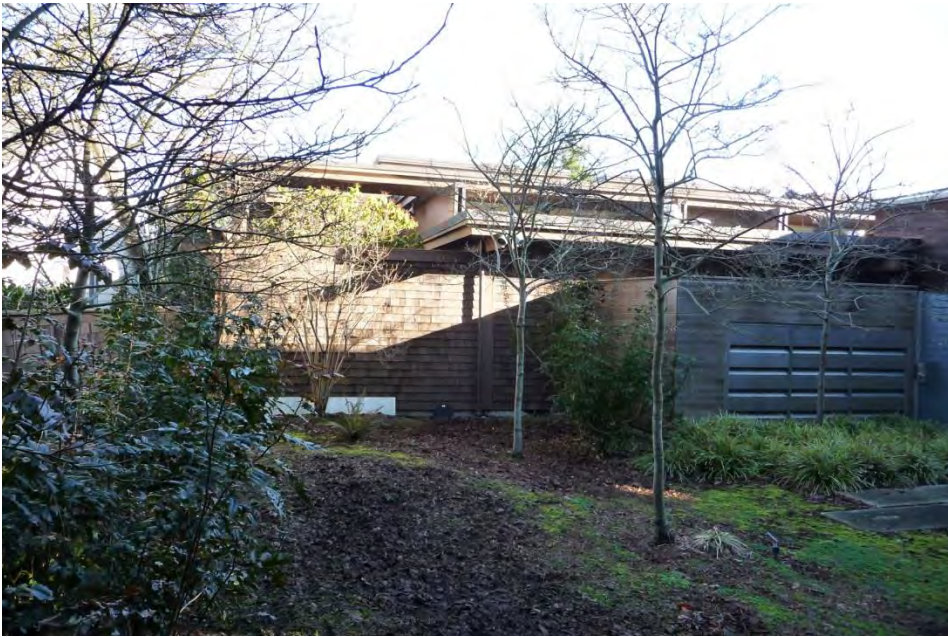
Photo #8 Exterior view, west facade, north end, camera facing east Photographer: Susan Boyle, January 14, 2015
