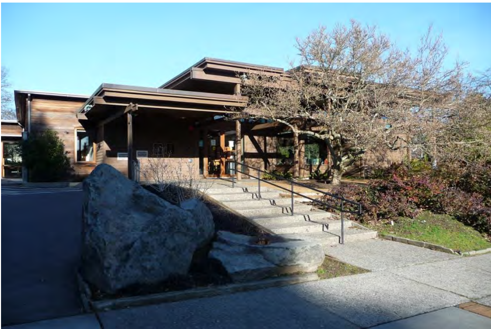
Photo #3 Exterior view of main entry, camera facing northeast Photographer: Susan Boyle, January 14, 2015
