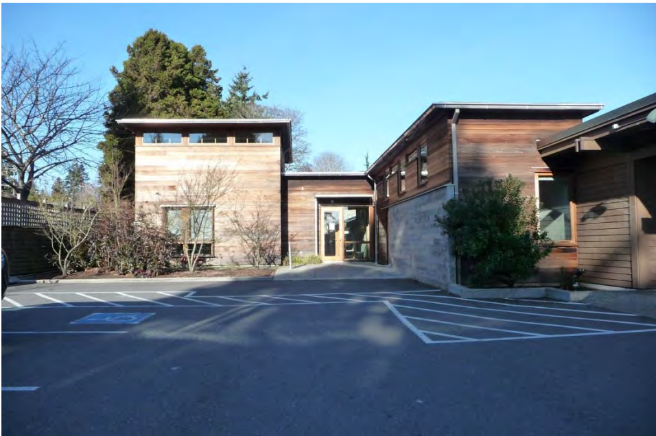
Photo #5 Exterior view, expansion and addition, camera facing north Photographer: Susan Boyle, January 14, 2015
