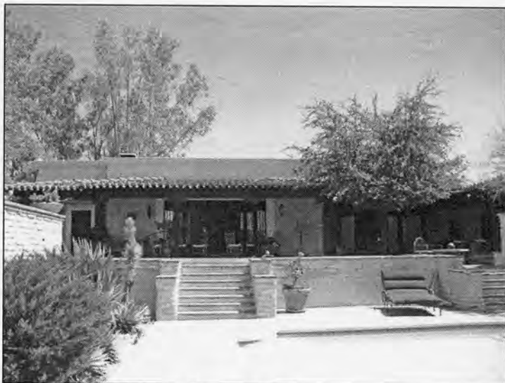
Photograph #3 South façade, camera facing north.
