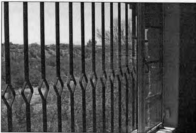
Photograph #7 Example of steel casement window opening with decorative iron grill work.
