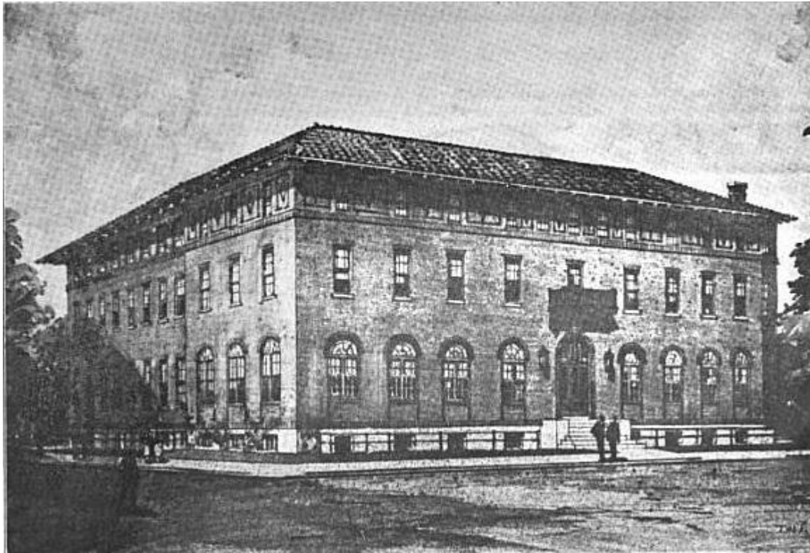
Figure 6: Rendering of the National Catholic Community House. Source: East St. Louis Journal , 1920.
