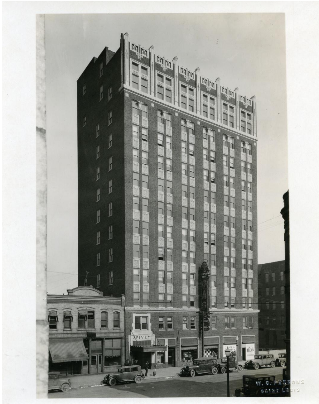
Figure 10: The Spivey Building upon completion in 1927. Source: W.C. Parsons Collection, Missouri History Museum.
