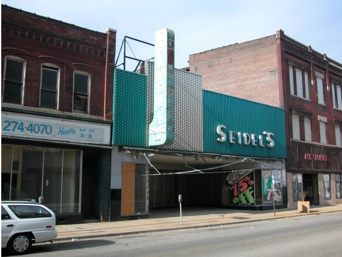
Figure 12: The Seidel's Apparel Company Building as it appeared in 2005. Note building at right that is no longer extant. Source: Michael R. Allen photograph.
