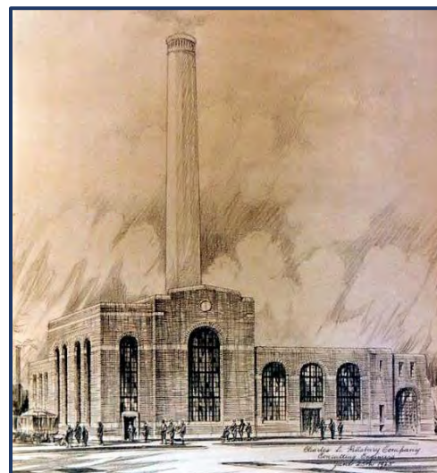
Electric, Light, Ice & Water Plant, 1925 (C.L. Pillsbury Co.)
